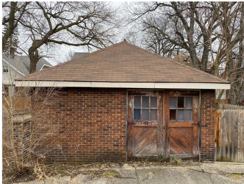
Garage (West elevation—restoring the carriage doors is on the future list)
