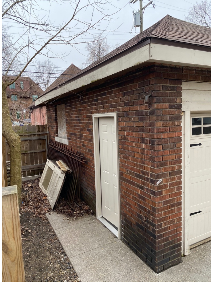
Garage (Southeast elevation)
