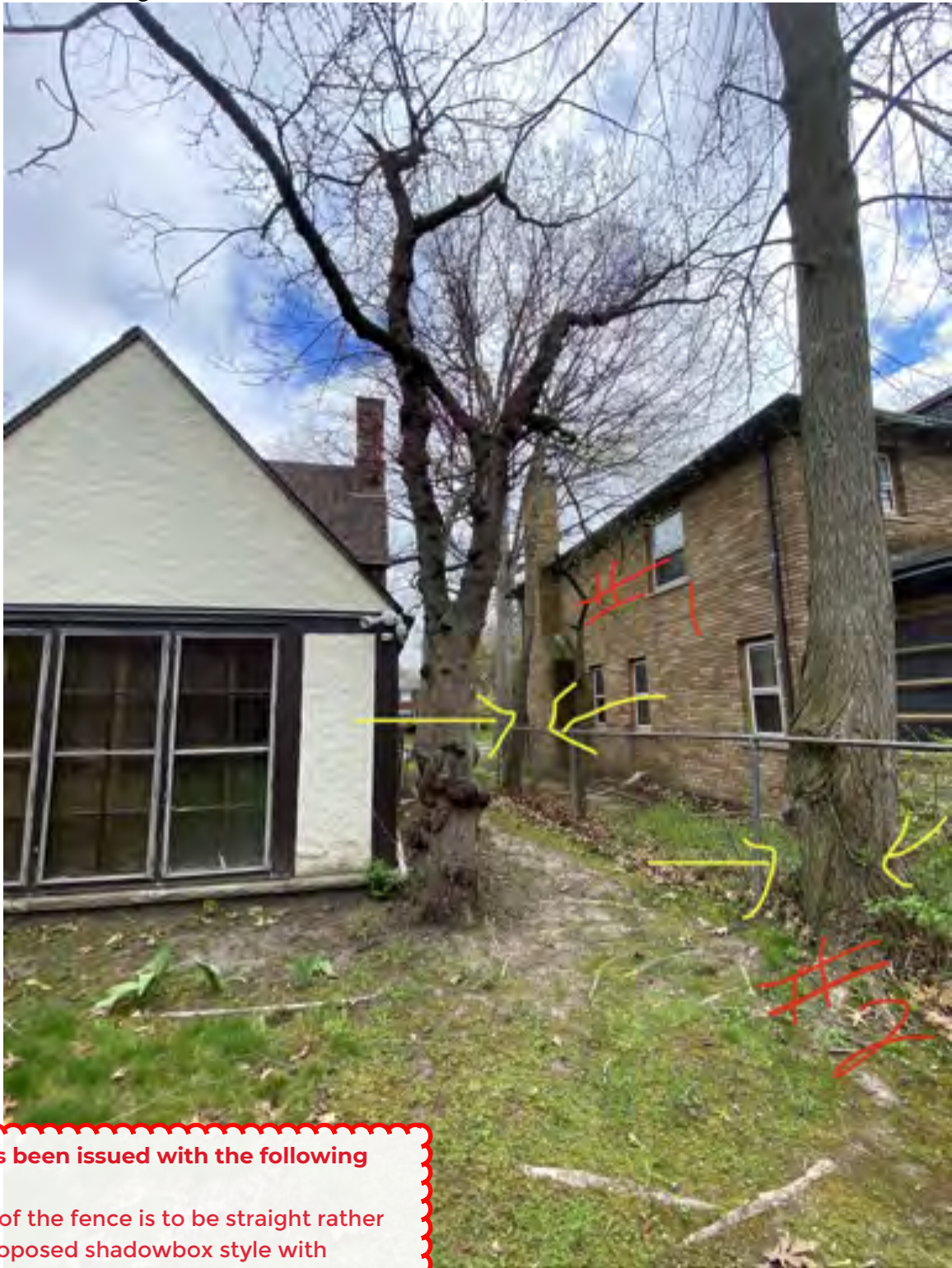
Trees needing removal for fence installation (east):
