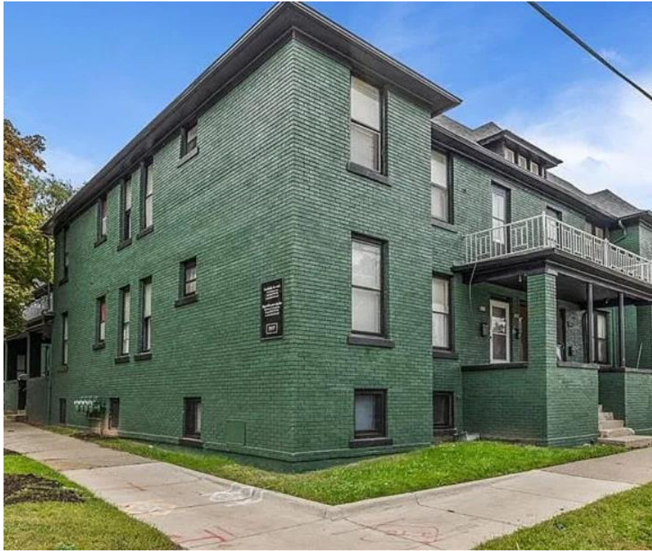
Existing building as viewed from the corner of Campbell and Toledo (looking southwest).
