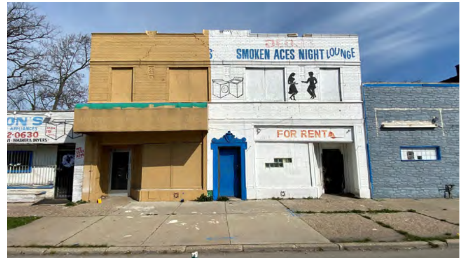
The Smoken Aces Night Lounge is the first property being targeted for stabilization and redevelopment through the Tactical Preservation initiative by the City of Detroit.
