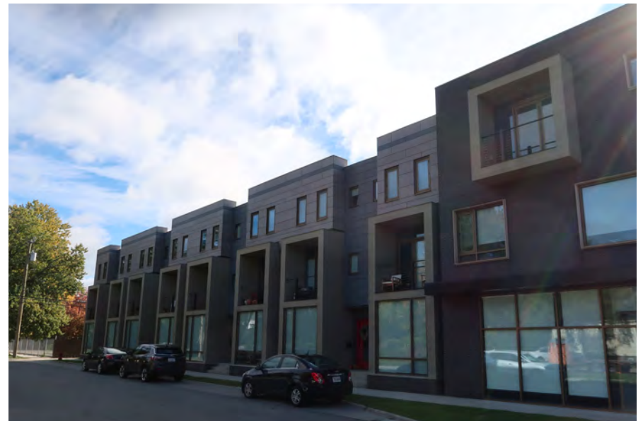
The Coe, a newly built mixed-use development in West Village
