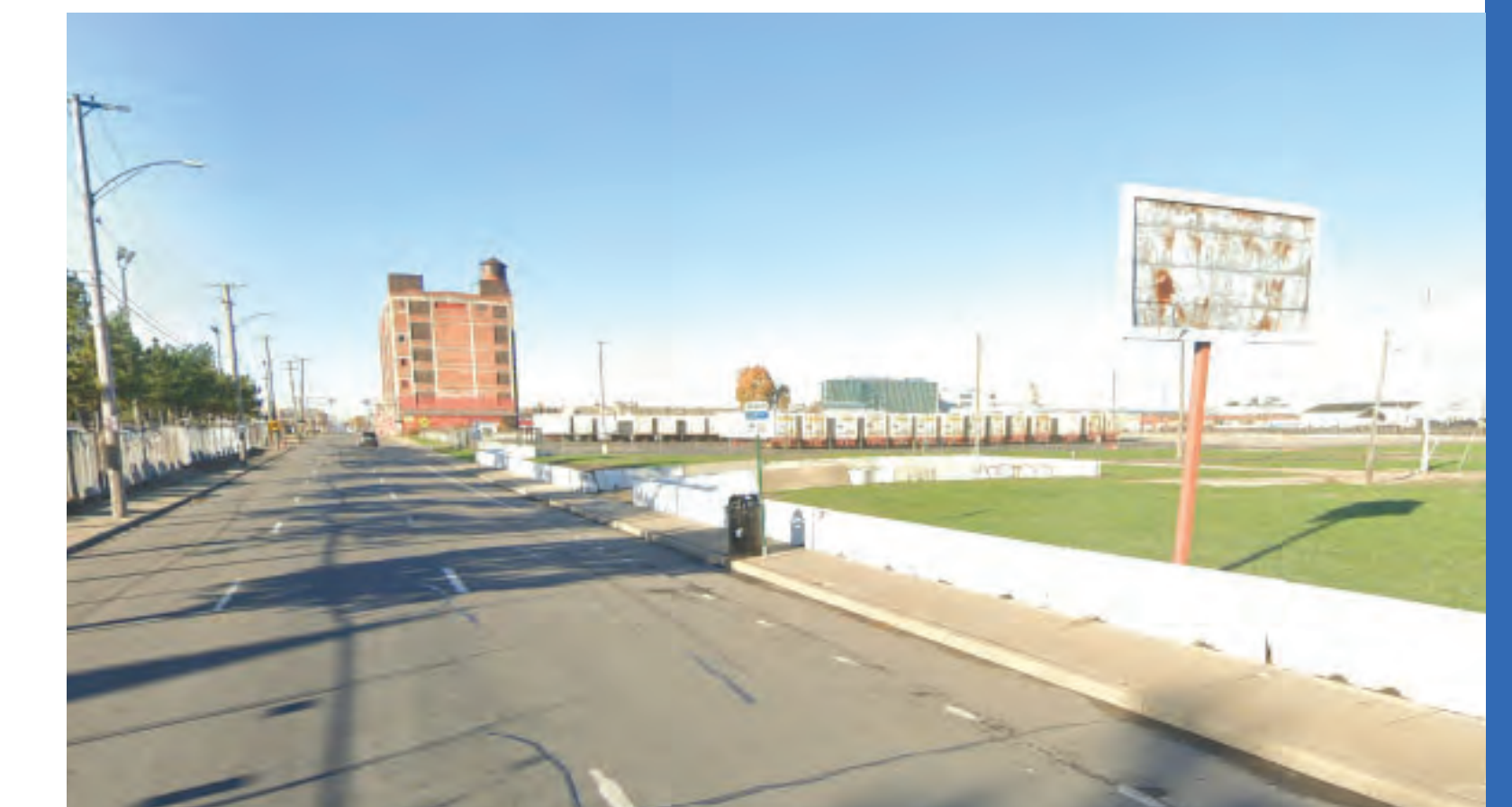
Potential for a mobility hub on the JLG where it meets Warren.
