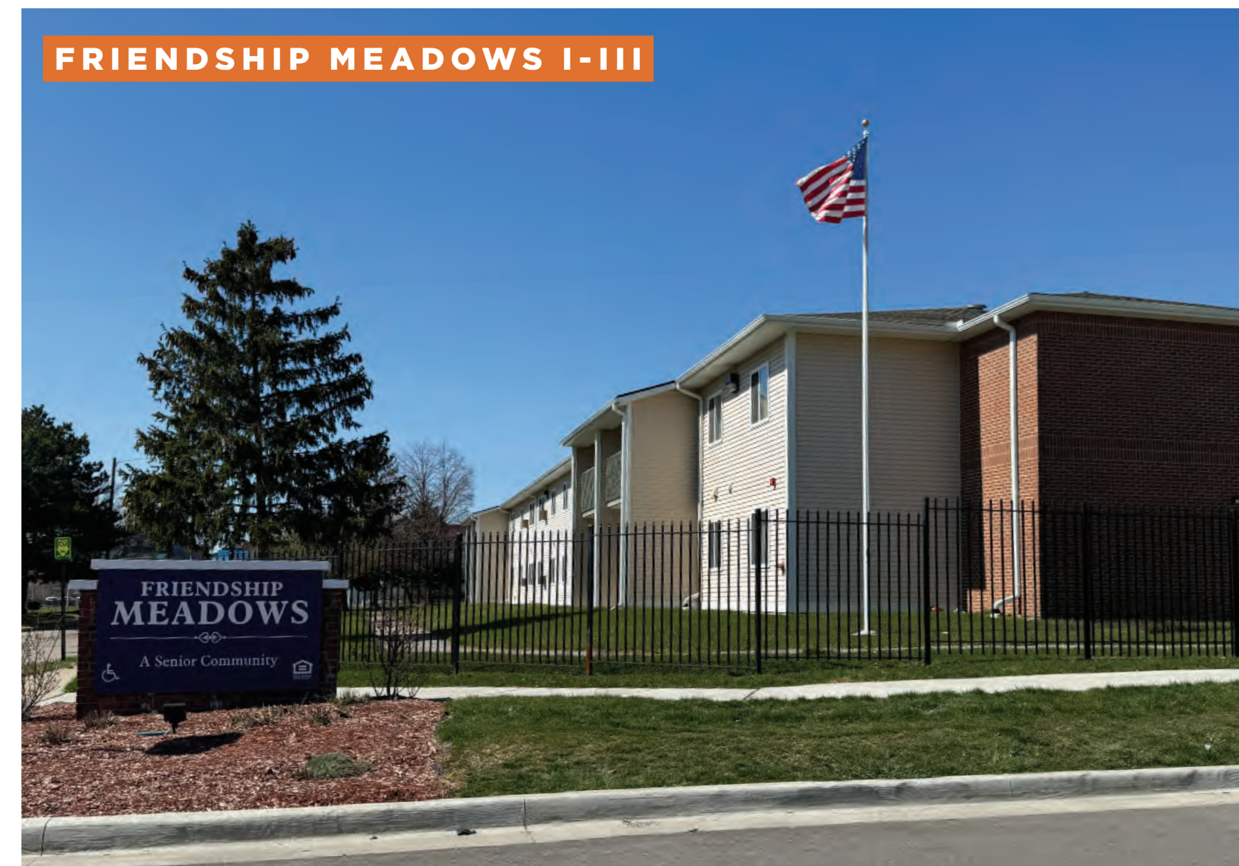
Between 2020 and 2022, Communities of Hope, Inc preserved and rehabbed 206 units affordable to those earning between 40% and 60% AMI at Friendship Meadows in the Forest Park neighborhood, through LIHTC awards.
