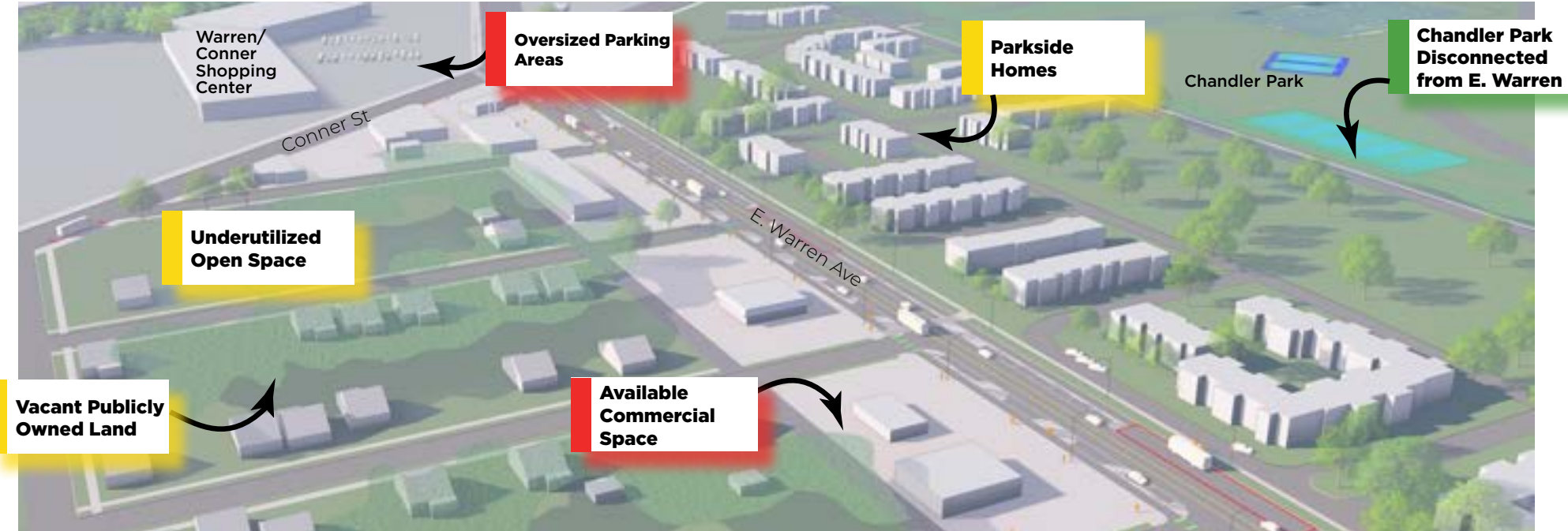
Existing conditions of E. Warren Avenue and Conner Street.
