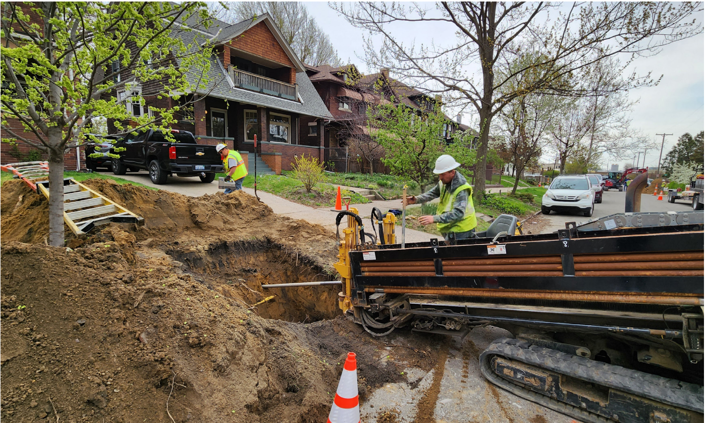
A DWSD contractor replaces a lead service line with copper.
