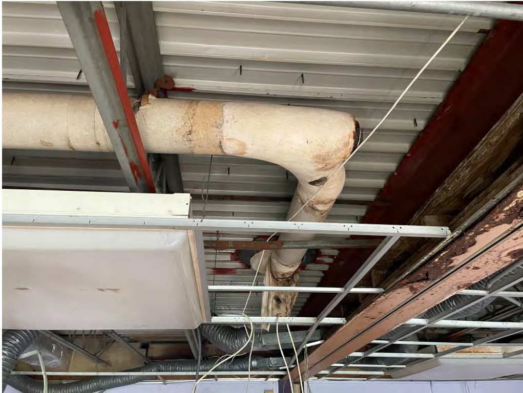
Roof drain pipe
