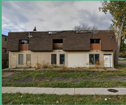
Demolishing Non-Historic Vacant Buildings
