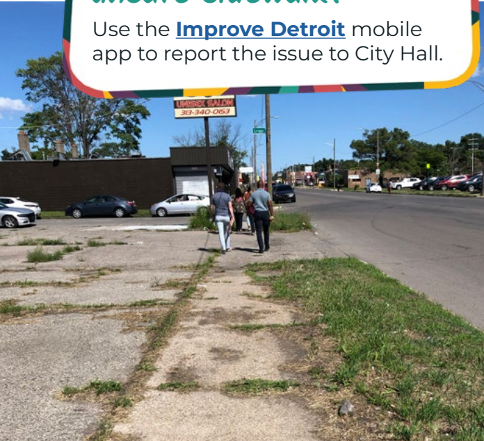
OVERGROWTH OF GRASS OR MISSING CURBS
