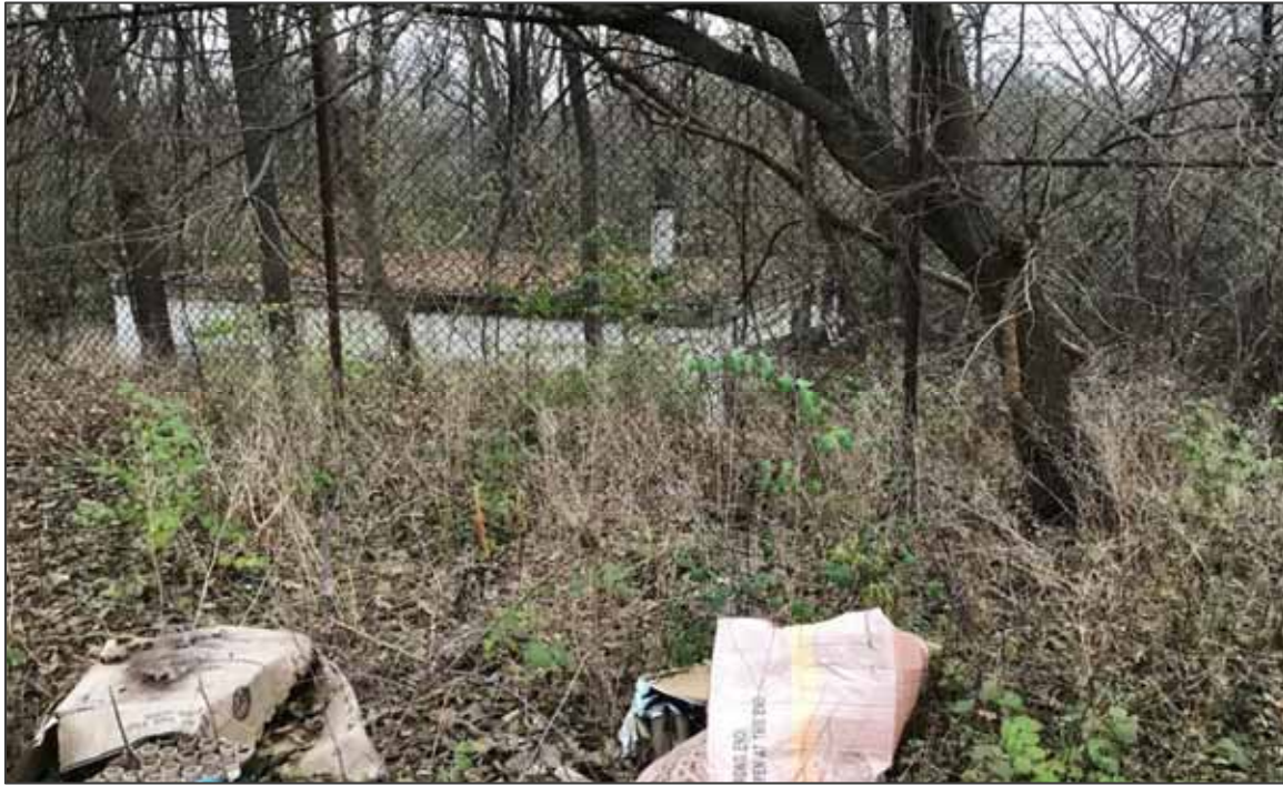
PHOTO NO. 25: View of the former refrigeration building within a fenced-in area northwest of the clubhouse.
