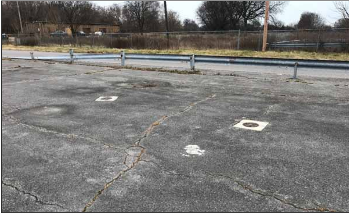
PHOTO NO. 23: View of two monitoring wells observed in the southern portion of the parking lot on the western parcel.
