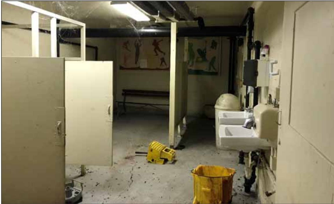
PHOTO NO. 39: View of the northern basement of the clubhouse.
