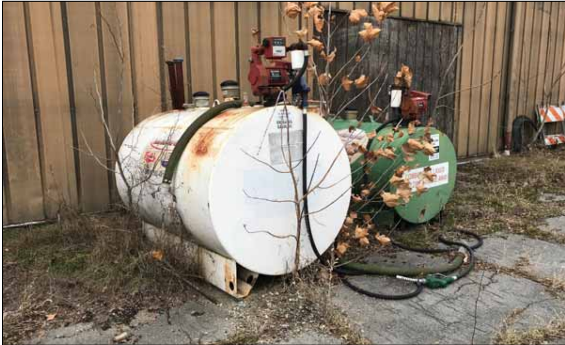
PHOTO NO. 3: View of a diesel and unleaded gasoline ASTs located south of the maintenance building.
