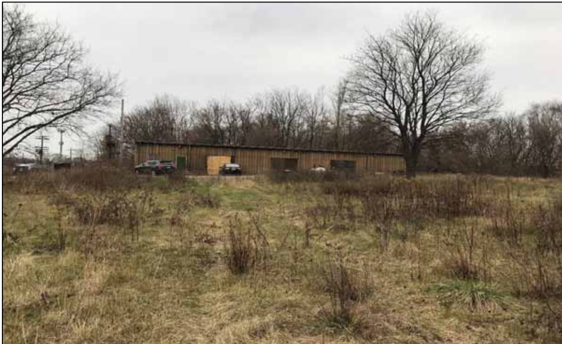
PHOTO NO. 2: View of the maintenance building located on the northwestern portion of the eastern parcel.
