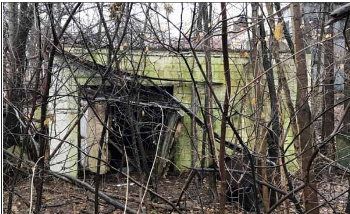
PHOTO NO. 32: View of the former refrigeration house, looking east.
