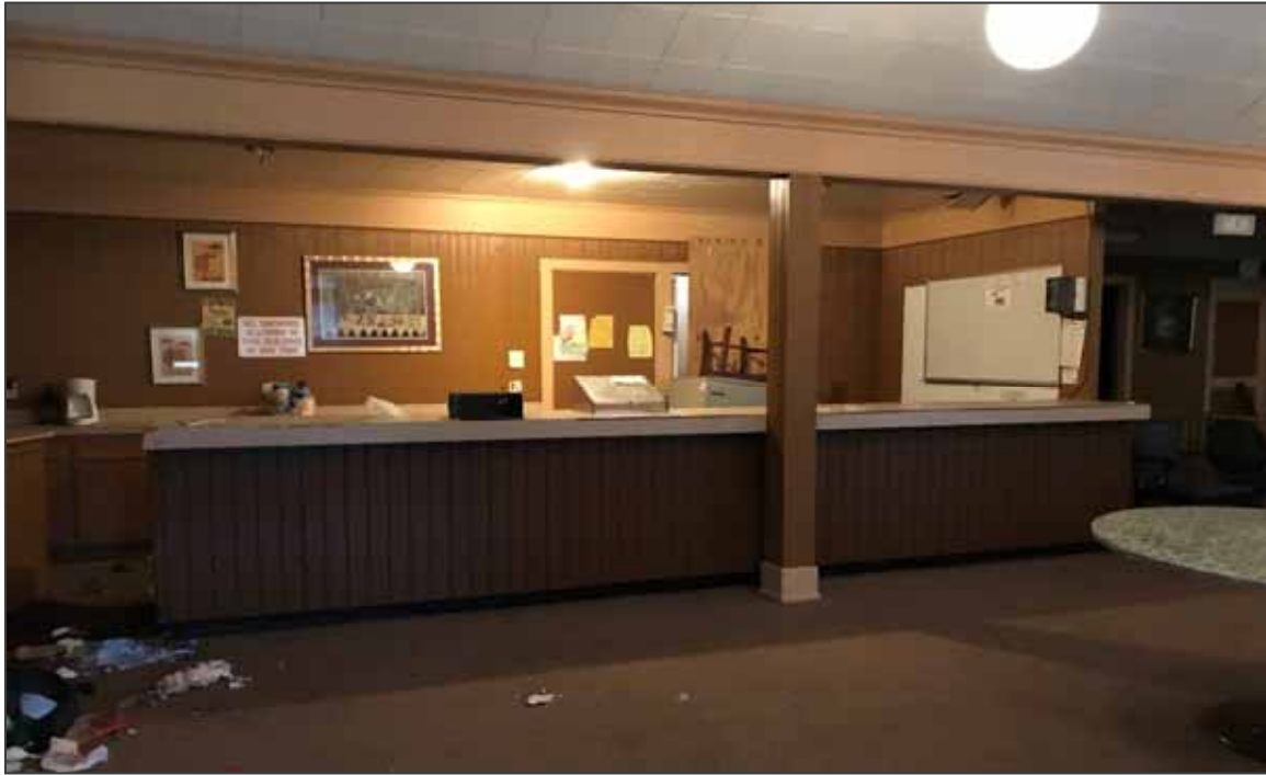
PHOTO NO. 37: View of the lobby of the golf course clubhouse.
