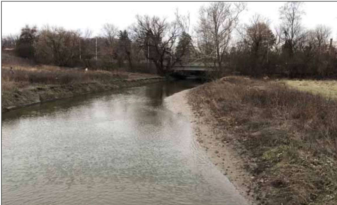
PHOTO NO. 30: View from the southern bridge on the southern portion of the western parcel.
