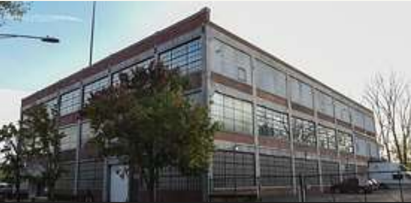
COMMERCIAL & INDUSTRIAL DEVELOPMENT
