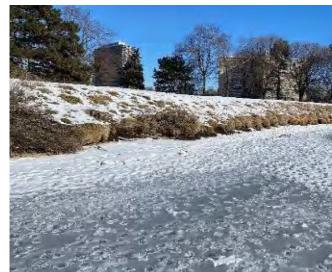
Noted erosion at berm section
