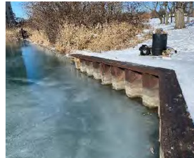
Steel sheet pile wall return
