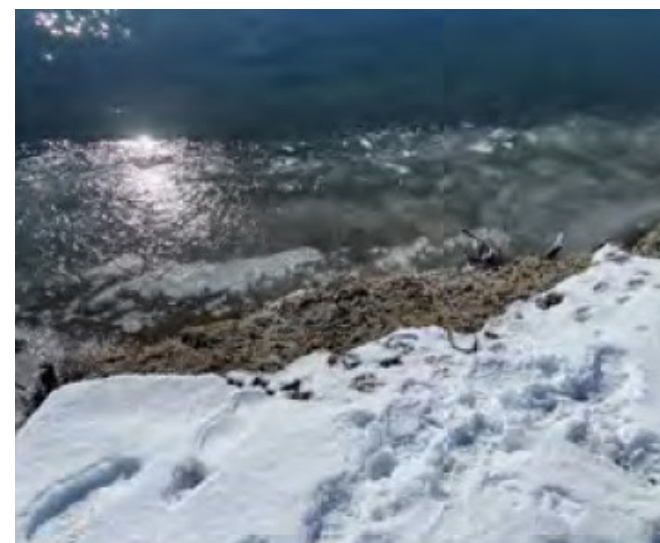
Unformed concrete poured along portions of shoreline
