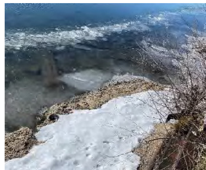
Unformed concrete poured along portions of shoreline
