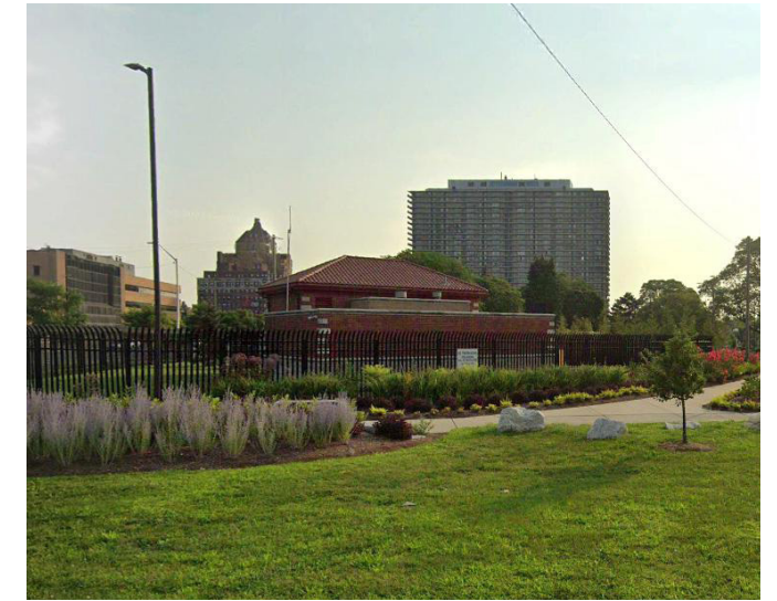
DWSD Pump Station and gardens near Jefferson Ave.
