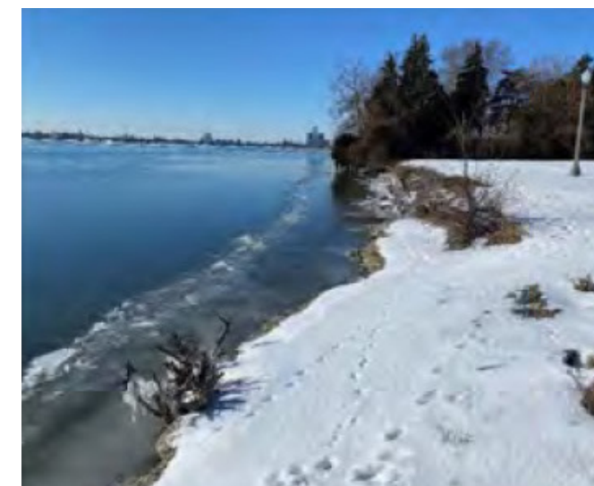
No shoreline flood protection, significant erosion observed
