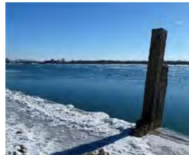
Deteriorated concrete structural component with exposed rebar
