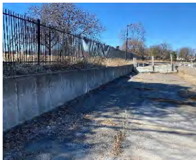
Concrete retaining wall is in good condition
