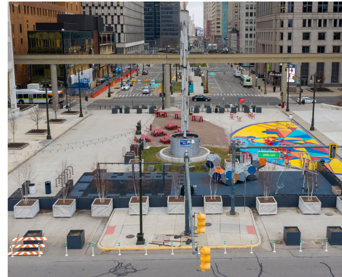
Planters and plastic delineator posts are placed along Jefferson Ave. to close Woodward Ave. to vehicles
