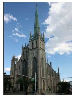
Fort Street Presbyterian Church Photo by Historic Detroit
