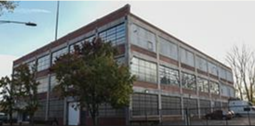
COMMERCIAL & INDUSTRIAL DEVELOPMENT
