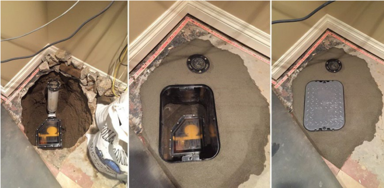
Installation of a backwater valve
