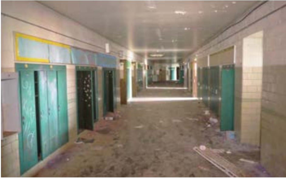
Second floor main corridor. showing finishes in relatively good condition.
