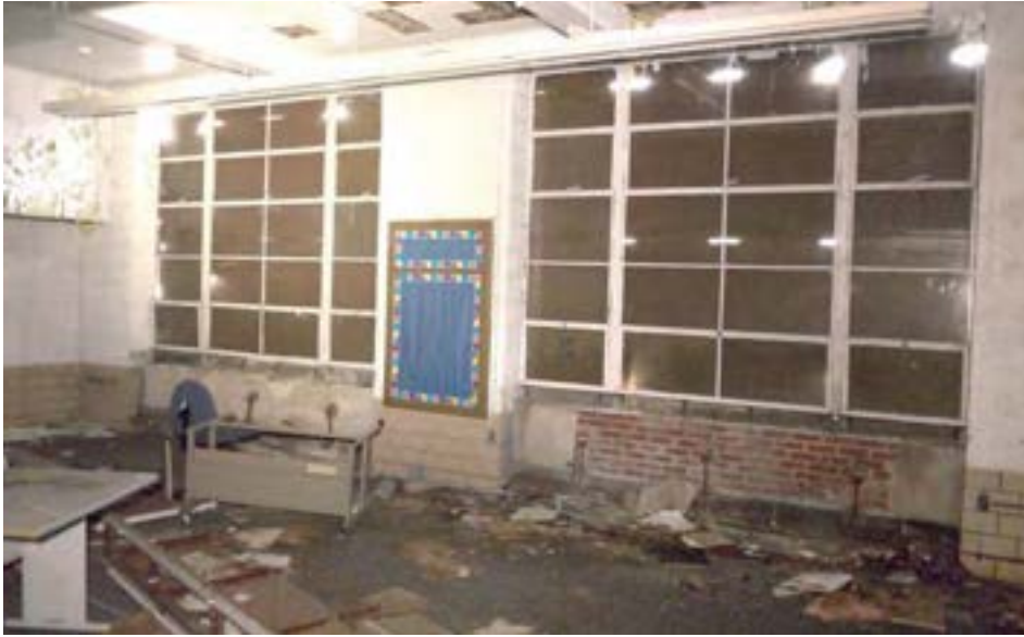
Classrooms feature large double windows consisting of a 4x5 steel-frame grid. Most of the original windows at Parkman remain intact.
