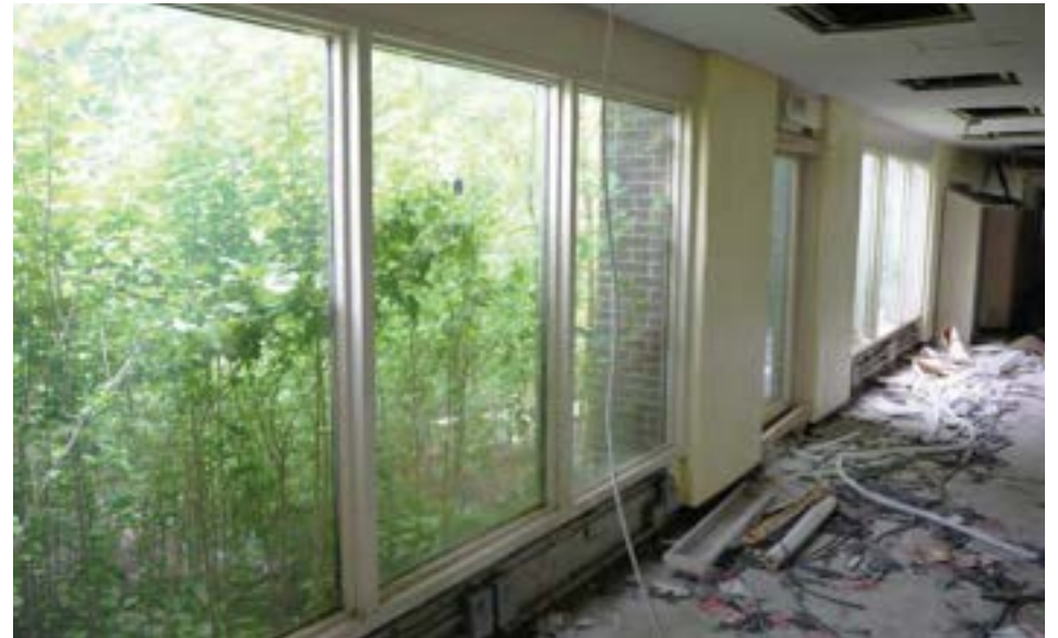
Courty contains two internal green courtyards. North-south corridors are single-loaded with classrooms on the outside, and windows to the courtyards on the inside.
