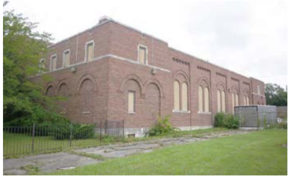
The large gymnasium wing viewed from southwest. The original arched window openings have been covered up with the same stucco panels as the classroom windows.
