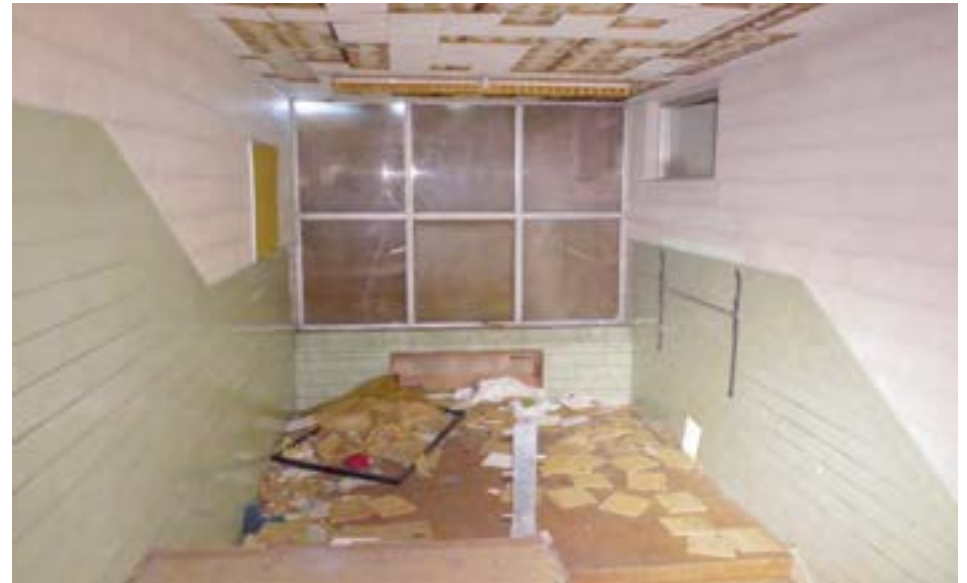
This stairwell features a spacious landing with large steel-framed windows that would have provided ample natural light and views to both first and second-floor corridors.
