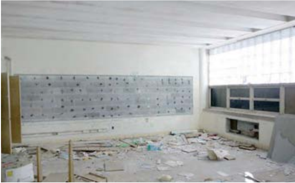
Classrooms are typical of 1950s-era schools, with concrete block construction, and wall-to-wall ribbon windows comprised of glass block over steel-framed operable lites.
