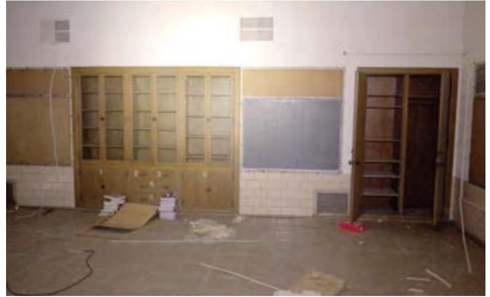
Classrooms feature simple and durable finishes: CMU walls, acoustic tile ceilings, VCT floors, and simple wood cabinetry.
