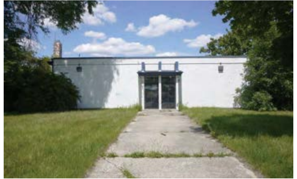
The southeast entrance facing Cathedral Street is a non-descript door with no embellishment. The single-story school is built on grade and has all accessible entrances.
