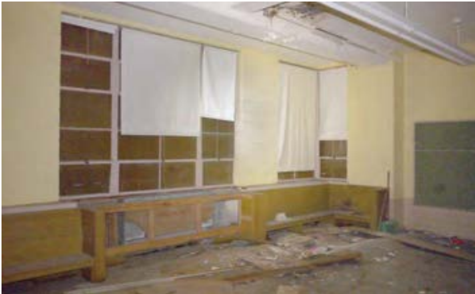
The kindergarten space dispenses with the deep 5-sided bay window that is a hallmark of Detroit elementary schools constructed during the 1920s and 30s. Instead, there is a rectangular alcove with a large central window and wrap-around corner windows.
