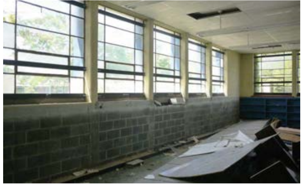
The library features the same steel-frame grid windows as the rest of the school, but they have been shifted higher to accommodate bookshelves below. The shelving in the foreground has been tipped over, but some standing units are visible at far right.
