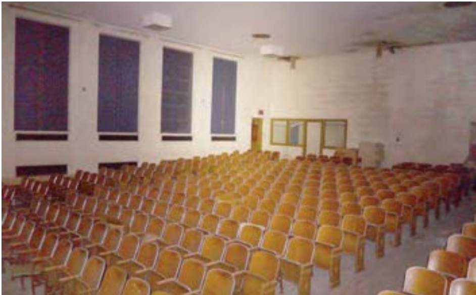
The auditorium, added in 1952, is a simple CMU box. Original wood seating and steel-frame windows are still intact.
