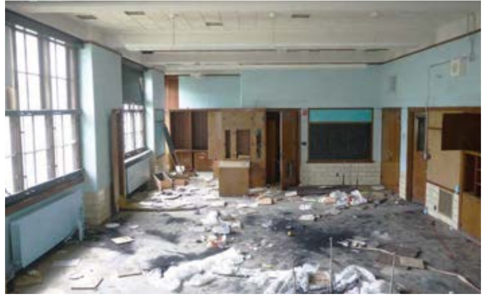
First floor "practical arts" classroom with intact windows and wood cabinetry.
