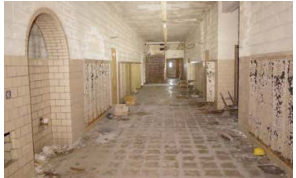
Interiors are simple and sturdy masonry construction, with glazed block accents. Arched alcoves once housed drinking fountains, which have been taken. The corridors do not receive much natural light; the only sources are narrow slit windows in the stairwells at the ends of each corridor.
