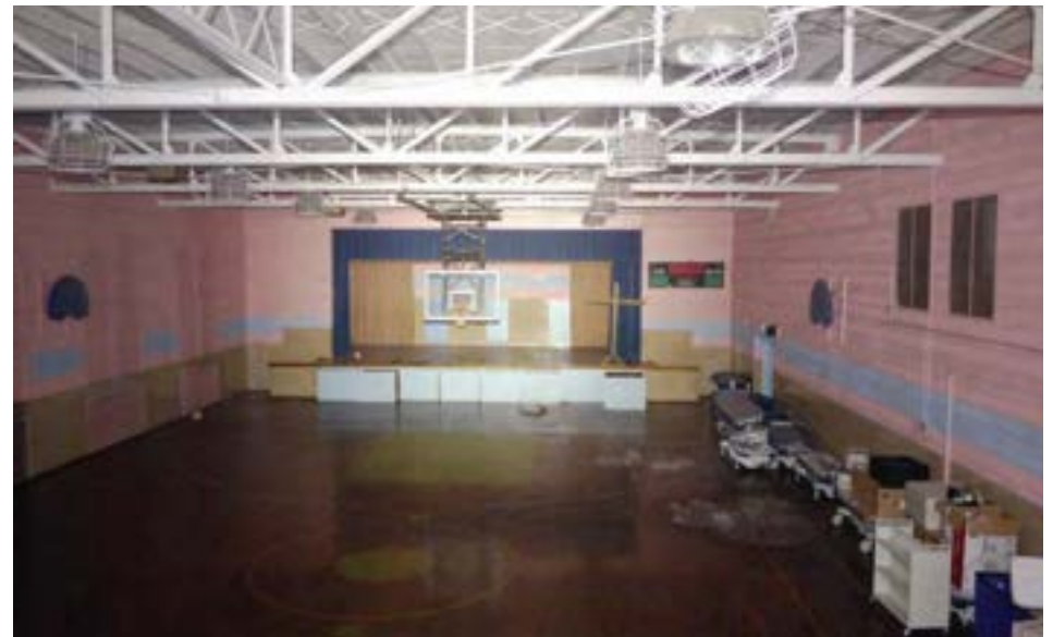
Gym and stage viewed from balcony seating. The gym's exterior wall was originally lined with pairs of tall arched windows, which were later filled in with CMU. These windows could be restored to flood this currently dark space with natural light.
