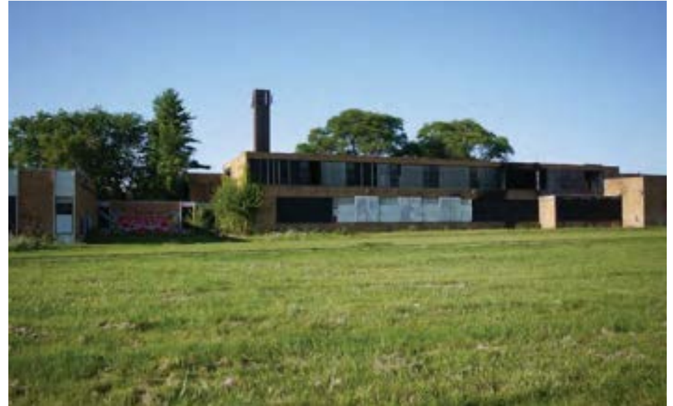
North elevation of the 1955 unit, viewed from Simanek Playfield. Strong horizontal lines typical of 1950s-era International Style school architecture. Smoke damage from first floor fire is visible at right.
