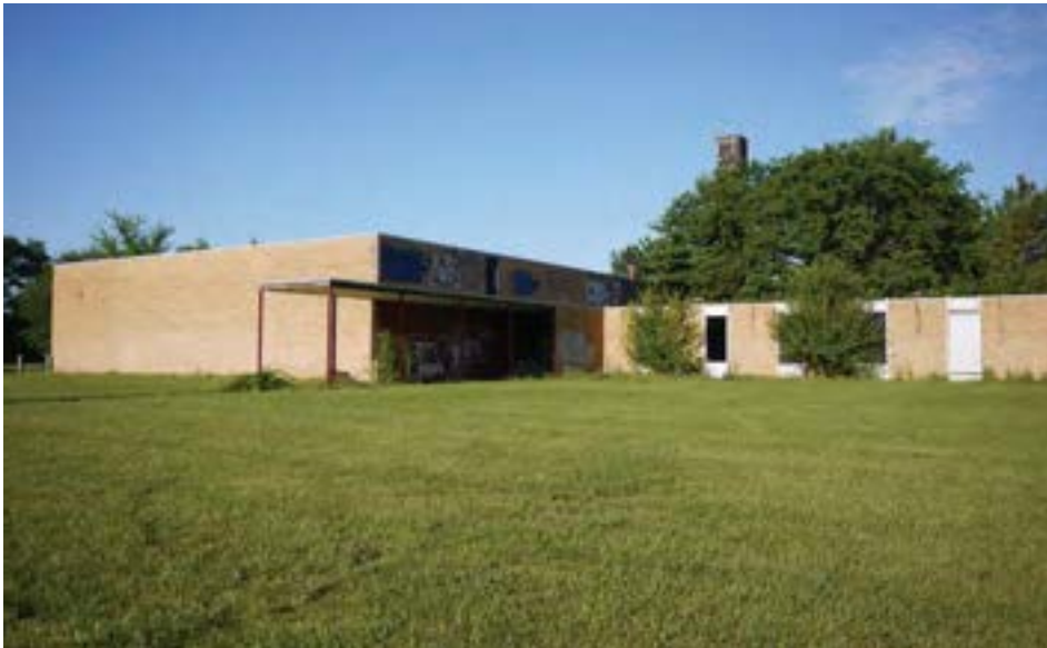
East elevation of 1963 unit viewed from Simanek Playfield. Large volume on left is the multipurpose cafeteria. Low volume to right is a connector corridor which provides a link to the workshop spaces and frames an interior courtyard.
