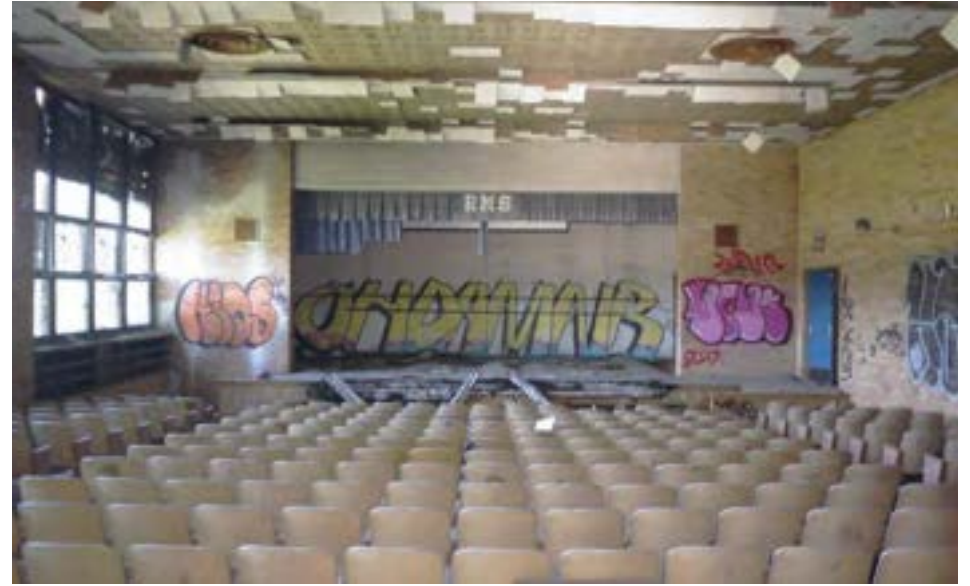
Brick auditorium in 1955 unit is in serviceable condition. Large grid of aluminum windows provides views to park; original design was presumably glass block.
