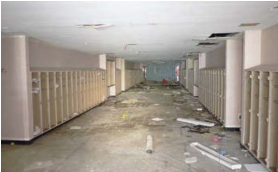
The main hallway is 17' wide with 8' ceilings and lockers lining the wall. The corridor forms a central axis between the main entrance and a decorative glazed tile art wall at the opposite end.
