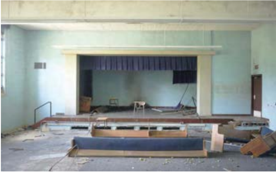
The small auditorium has a low and wide stage area and a flat floor. Its finishes are simple painted concrete.
