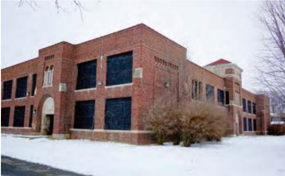
The southwest and southeast (front) elevations of the school showcase the building's decorative brickwork and distinctive entryways.
