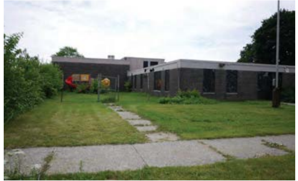
North elevation showing small playground with main classroom building at right and larger gym/auditorium volume in background.
