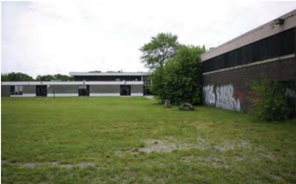
Biddle is located on same site as Sampson-Webber Elementary/Middle School, a large active DPSCD school (background). Biddle's gym is visible at far right. The two schools are separated by a shared service driveway.
