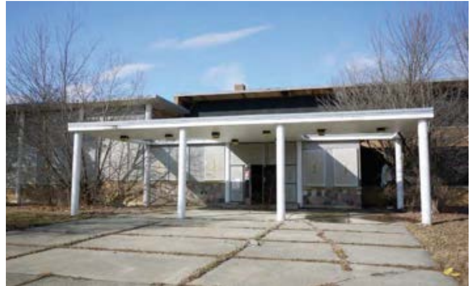
Koskiusko's main entrance is covered by a concrete canopy with two punched openings.
