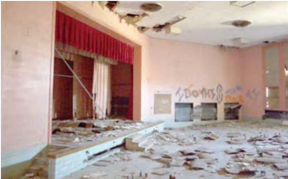
The 1951 auditorium features an unusual diamond-shaped configuration. The main seating area is a square space that is orthogonal to the rest of the school building, while the stage area is located in the corner and oriented at a 45-degree angle.
