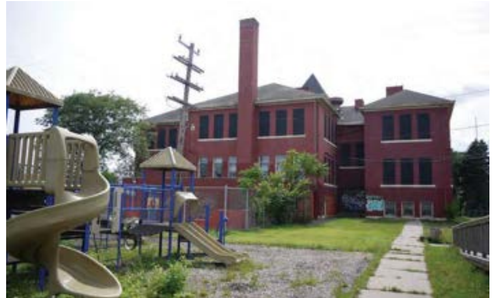
East (rear) elevation, with playground equipment in foreground obscuring 1900 boilerhouse addition.
