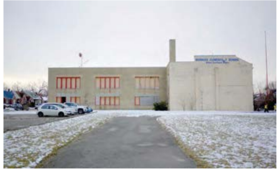
North elevation viewed from the school's asphalt track. The blank facade on the right of the image is where a 1973 addition once connected to the original building; the addition was demolished in 1991 or 92, according to Sanborn maps.
