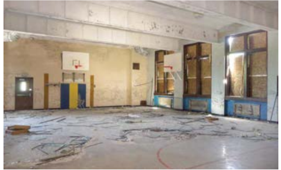
The gymnasium is in good shape, and appears to have been in use recently—debris has been swept away from beneath the basket. There does not appear to be water damage, and the floors have not bowed like most other gyms observed in this study.
