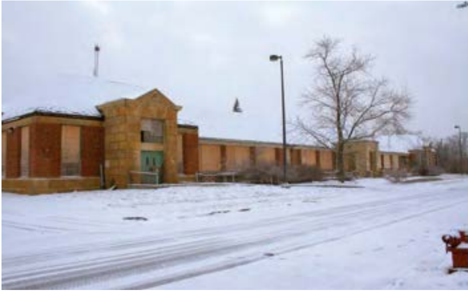
Oakman's west elevation viewed from the northwest corner. The nearest visible entrance on the left leads to the auditorium. One of the four primary school entrances is visible in the center of the building, marked by a stone portico.
