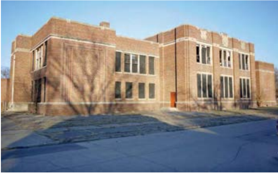
The exterior of the building features stone cartouches depicting academic, athletic, and Michigan themes. The facade also features multicolored diamond-pattern brickwork and limestone and formed-stone window frames. The 1928 addition is pictured above.
