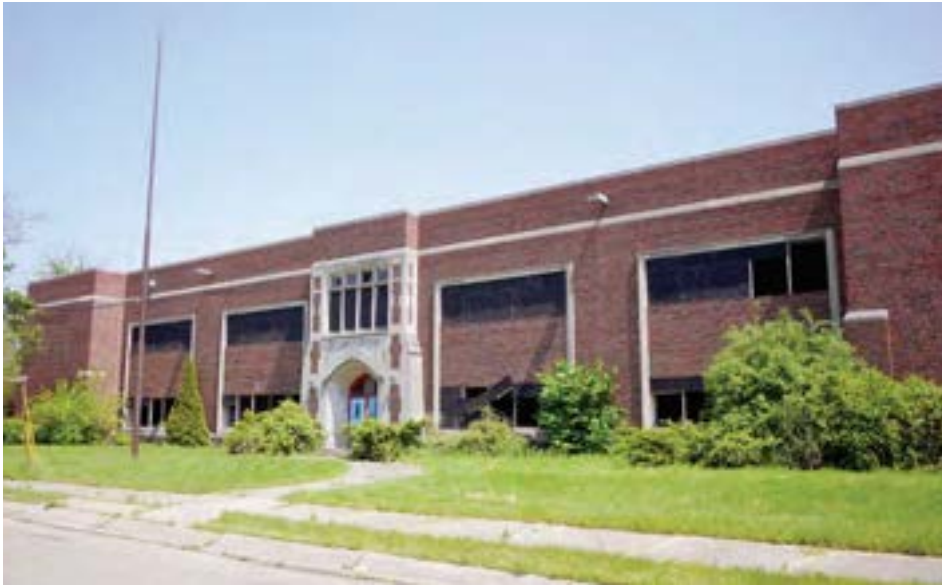
The facade is simple, with little ornamentation beyond the frame-like cast-stone details around the windows and at the parapet. The facade was modified at some point to reduce the classroom windows to horizontal bands.
