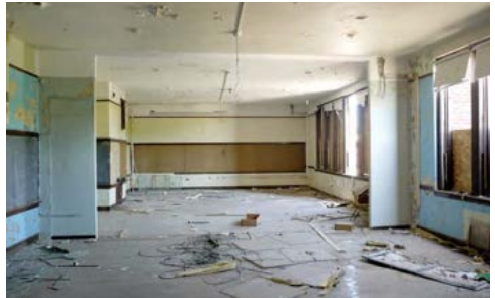
Two second-floor classrooms have been turned into one long room by removing the partition wall.
