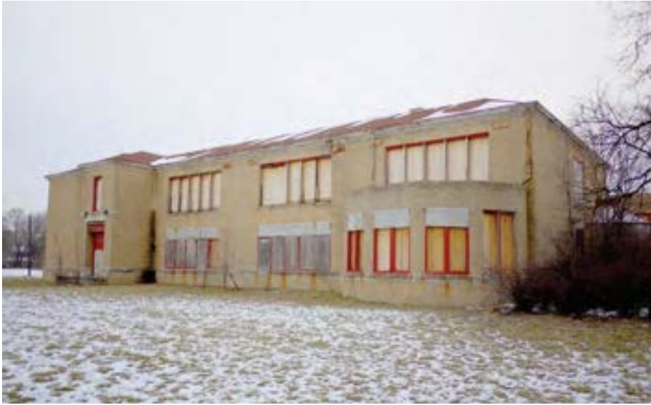
South elevation, with kindergarten bay window visible on the right side.
