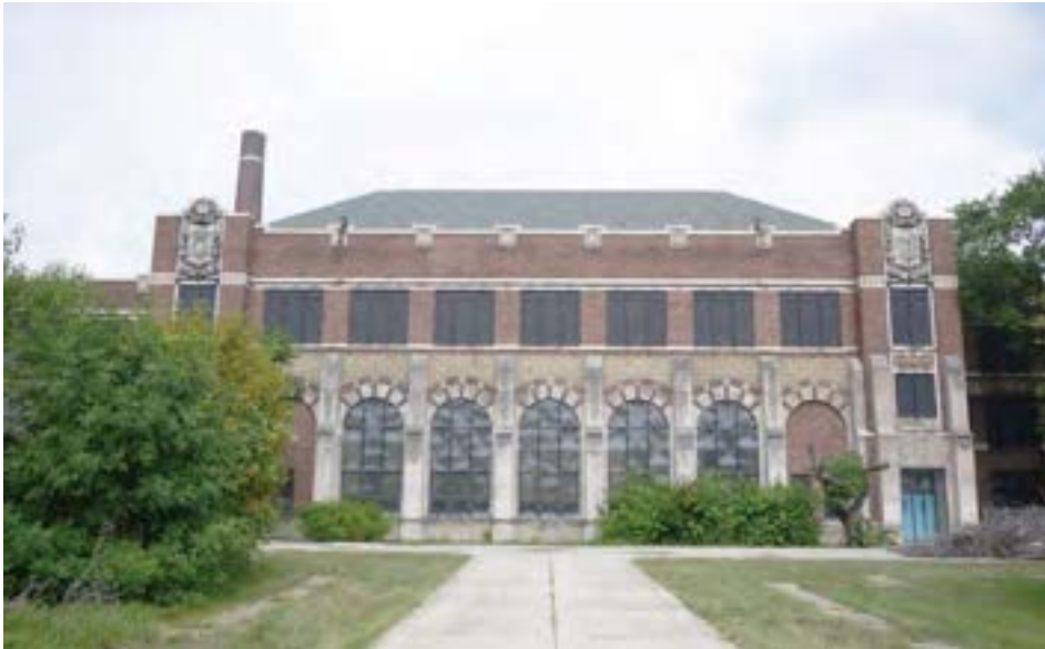
The west (main) elevation is dominated by the large arched windows of the auditorium. Two main entrances flank the auditorium, topped with elaborate stone ornaments.
