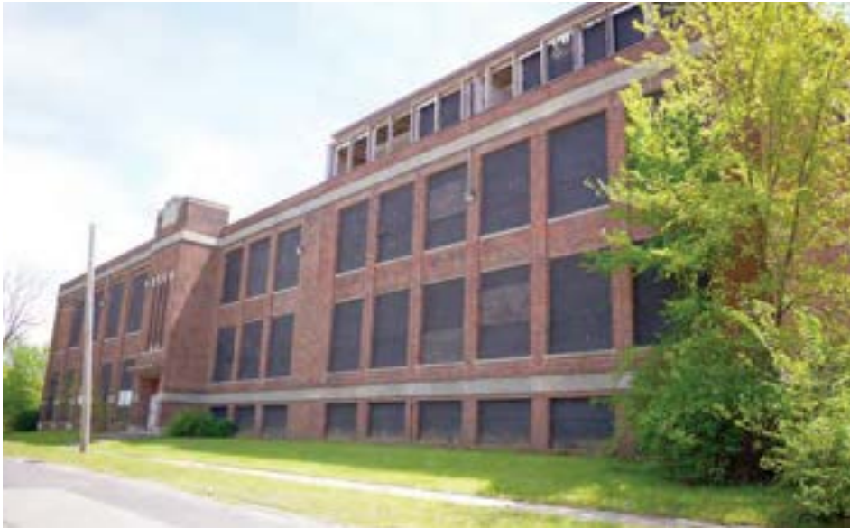
North elevation looking east. The wood-framed penthouse addition is visible above the roof of the original building. The gym and auditorium are at far left.
