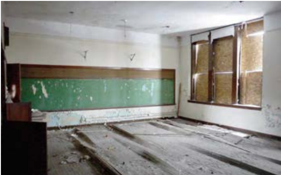
A typical classroom with plaster finishes in fair condition. The original wood-framed windows are missing throughout the school, and wood floors are buckled throughout.
