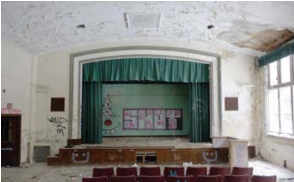
The auditorium features a suspended barrel-vaulted ceiling.
