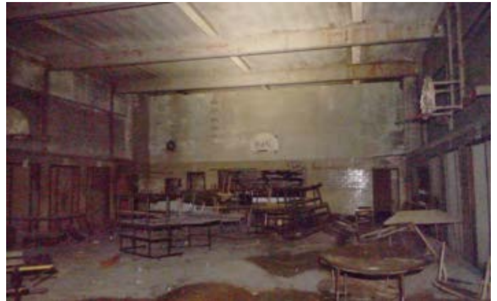
The 1951 gym is a windowless CMU box. Historic floorplans show that there were originally windows on both the north and south walls (presumably glass block matching the classroom addition). These windows were filled in with brick and CMU at an unknown time.
