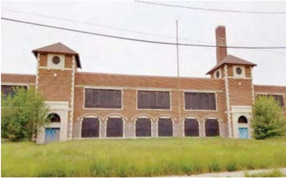
The long front elevation is symmetrical and anchored in the center by two entrance towers with hipped roofs.
