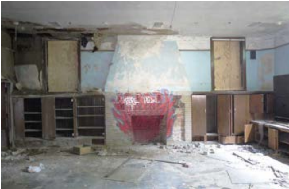
The kindergarten features a large brick fireplace, built-in wood cabinetry, and windows on multiple exposures.
