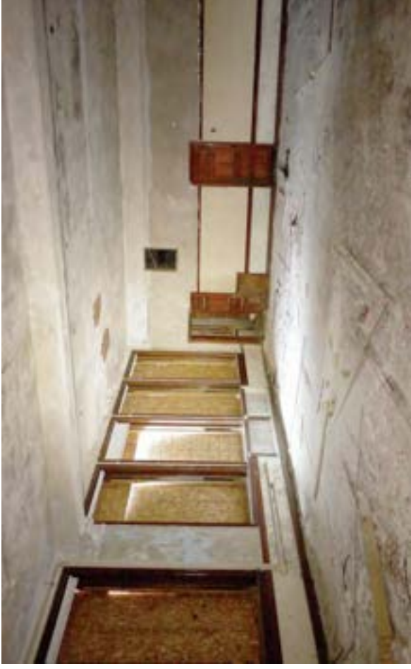
The kindergarten windows. Finishes in classroom areas were in generally good condition.
