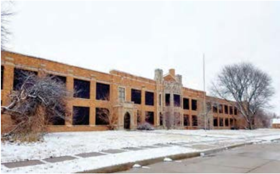
View of the front (south) elevation from Elmira St. The majority of classrooms are arranged along the south elevation.
