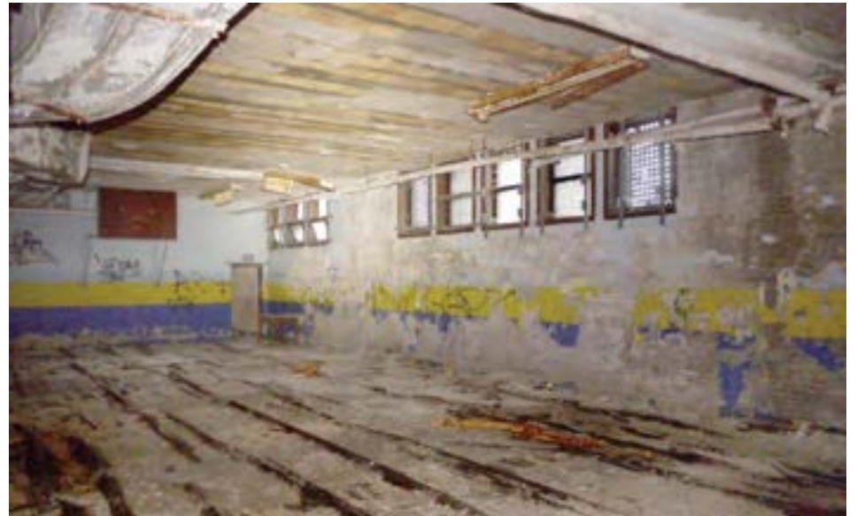
The basement-level gym is both longer and narrower than typical elementary school gyms. It is sunken four feet lower than the rest of the basement to achieve thirteen-foot ceilings.
