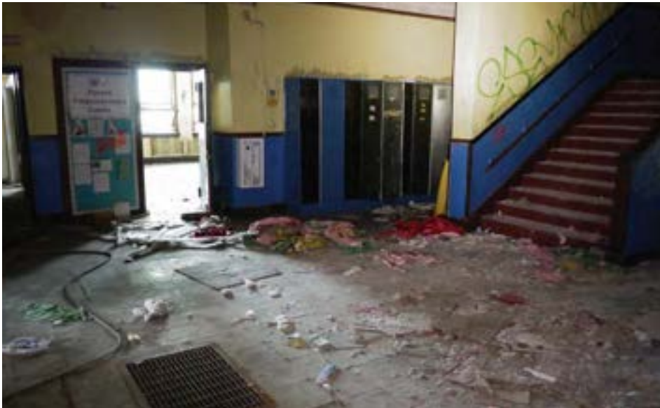
First floor main corridor in the original 1918 unit. Corridors have large landing areas at each end that serve the stairs and multiple classrooms.
