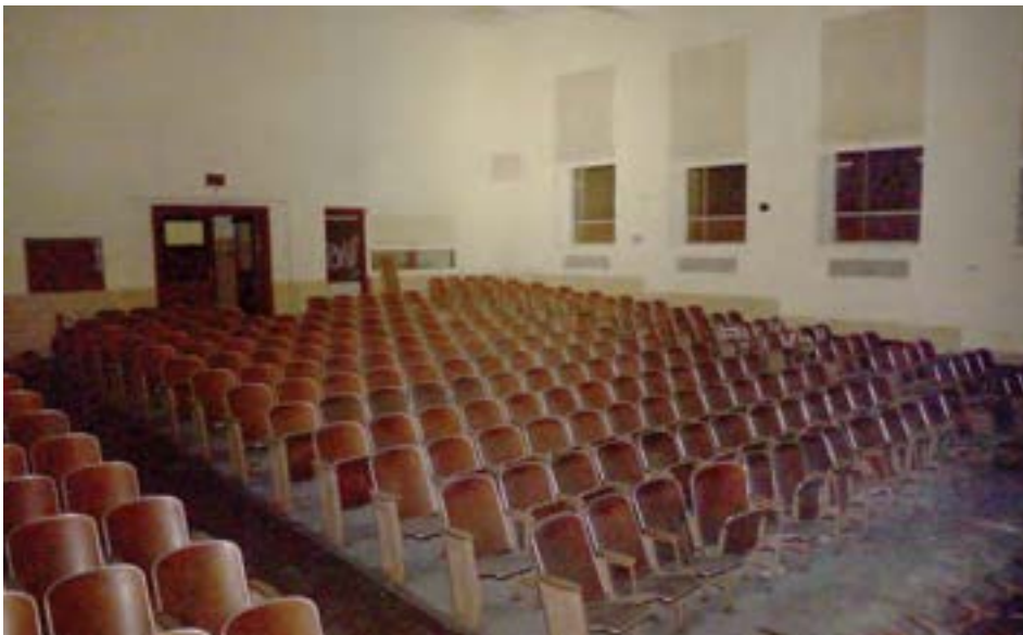
The auditorium is utilitarian CMU construction with no frills. While it is not a particularly beautiful or impressive space, it is solidly built and in relatively good condition. There is a dedicated entrance with vestibule and covered sidewalk near the street.
