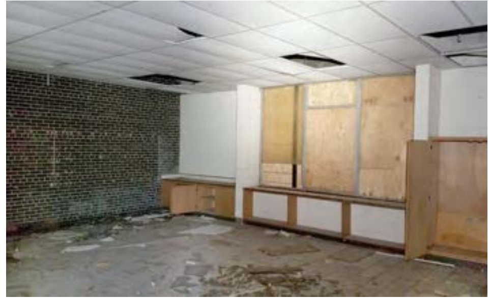
A typical classroom in the 1964 west addition. Newer classrooms feature smaller steel-frame windows in contrast to the wall-to-wall glazing that appears in the original classrooms. Here, the coffee-colored brick that clads the exterior facade reappears as an interior finish.
