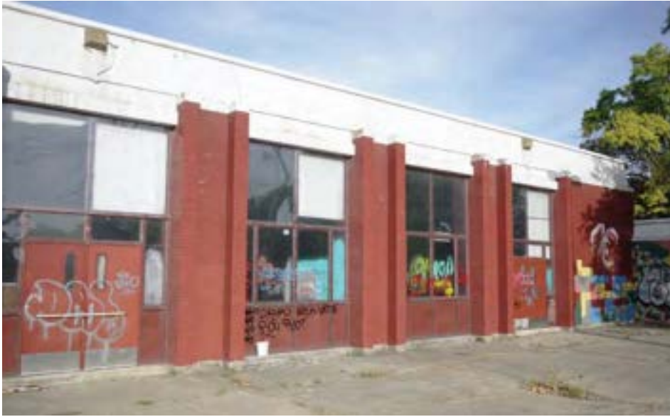
The eastern facade of the 1963 addition, showing a modern design with large storefront window systems. This view shows the large "cafetorium" space, which has multiple sets of doors leading out to a paved parking area.
