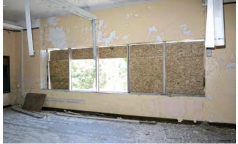
Classroom windows were partially filled in, leaving low strips instead of the usual tall openings seen in schools of the same era. The modern aluminum replacement frames have been scrapped throughout.
