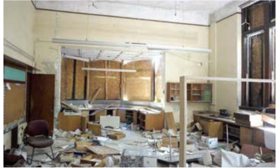
The first floor science room in the 1923 (south) wing includes a fully-enclosed conservatory and 16' tall ceilings.
