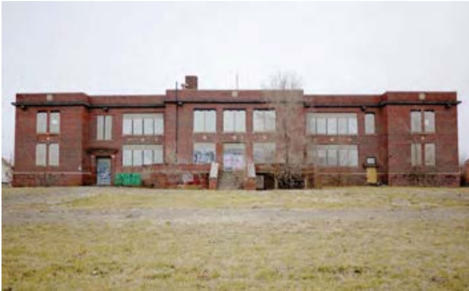
Rear elevation seen from the school yard. The stairs in the center of the building lead to a large outdoor terrace with access into the school's former kindergarten.
