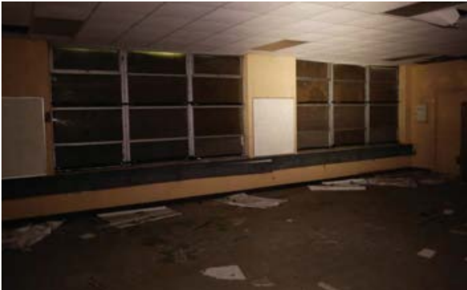
Typical classroom window configuration, with aluminum-frame lites with operable panels.
