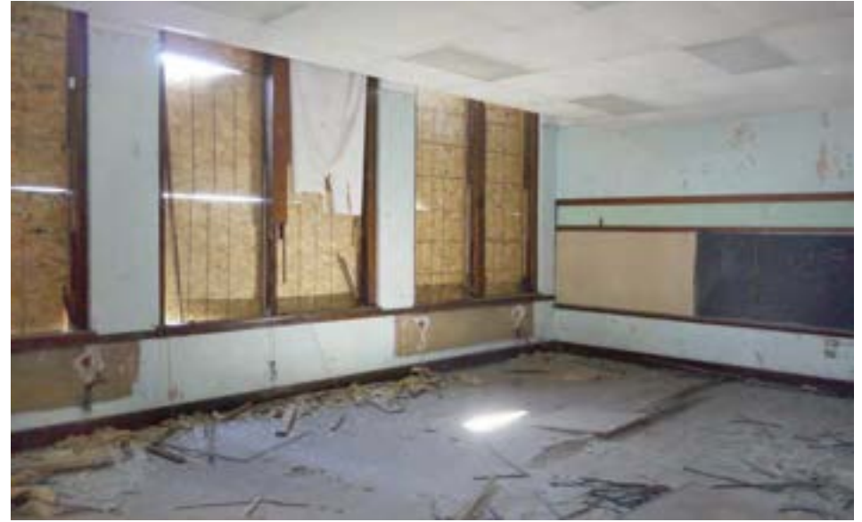
A typical classroom in good condition. Although the windows and radiators have been scrapped, the condition of the finishes is still good.
