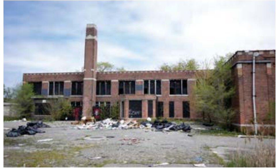
The rear (west) elevation of the school viewed from the parking lot. The entire classroom wing with kindergarten bay is visible, with the gym protruding to the right of the frame.
