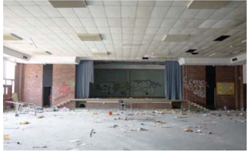
The stage area of the 1963 multipurpose "cafetorium." This wide-open column-free space is approximately 70x70' with 16' ceilings and exterior access. It is brightly lit from a row of east-facing storefront windows.
