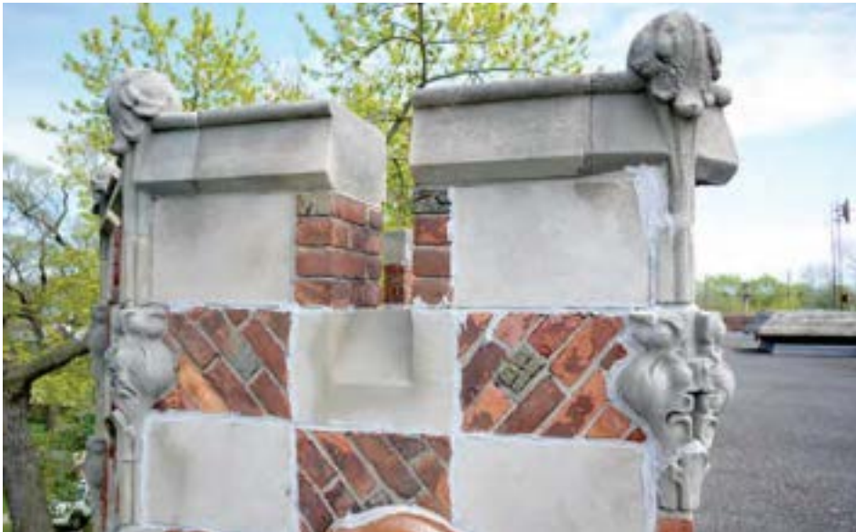
A closer view of the crenelations on the front towers reveals finely detailed cast stone embellishments and diagonal brick work.
