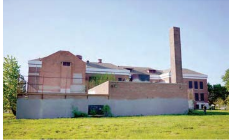
The rear of the school, with the 1962 gym addition in the foreground. The gym is built below grade and is connected to the basement level of the original building.
