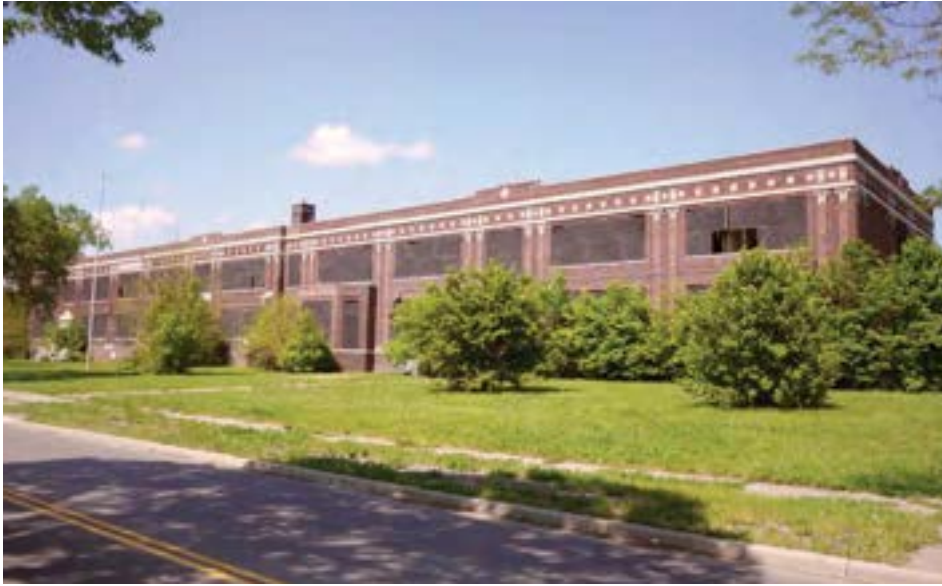
The main/west elevation, with 1923 unit in the foreground, and 1916 unit to the far left of the frame. Although the structural systems of the two wings is different and the two units have different floor heights, care was taken to preserve a unified appearance on the exterior.
