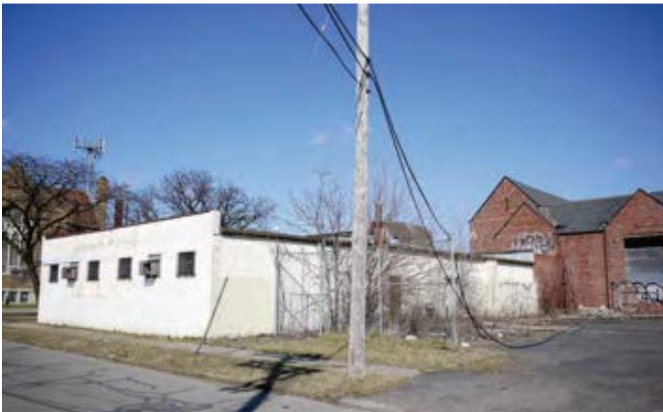
A 1950s-era commercial building adjacent to the school (formerly a commercial printer) was annexed by the school and connected to the gym.
