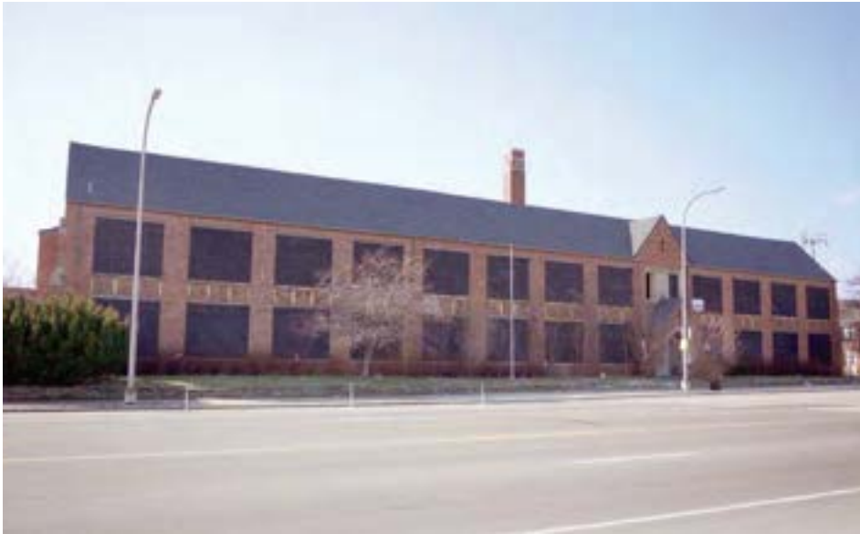
East elevation as seen from Livernois. While most schools have open space between the building and the street, Ruthruff has very small setbacks along Livernois and Chicago to the north.
