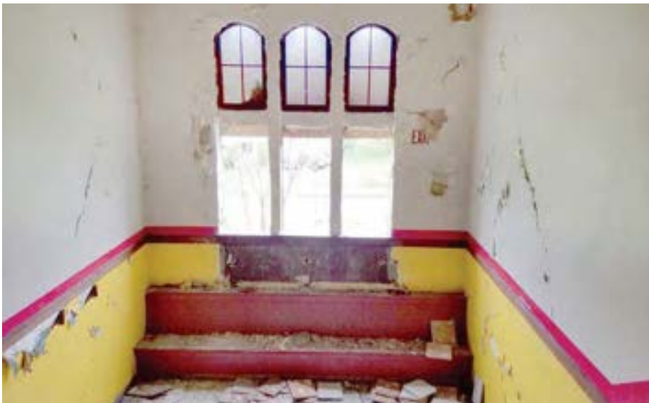
The north stairwell features arched windows and a wooden bench in the landing.
