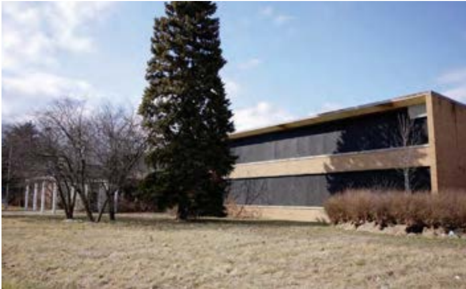
The front elevation viewed from the southeast corner of the building. The main classroom wing is a double-loaded bar featuring continuous glazing along its entire length. The white-columned canopy over the main entrance is visible at the far left.
