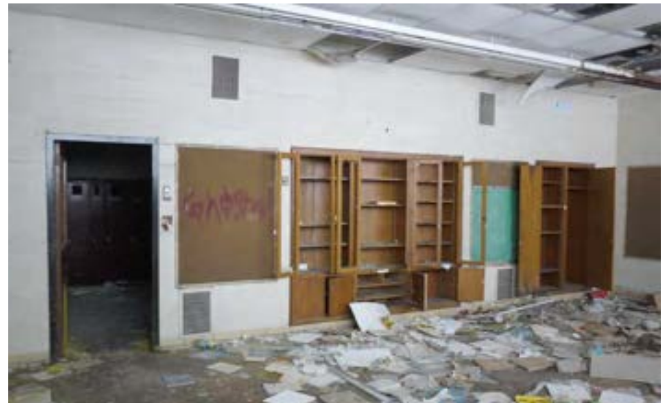
Built-in casework and other finishes in the 1951 classrooms are in good overall condition.
