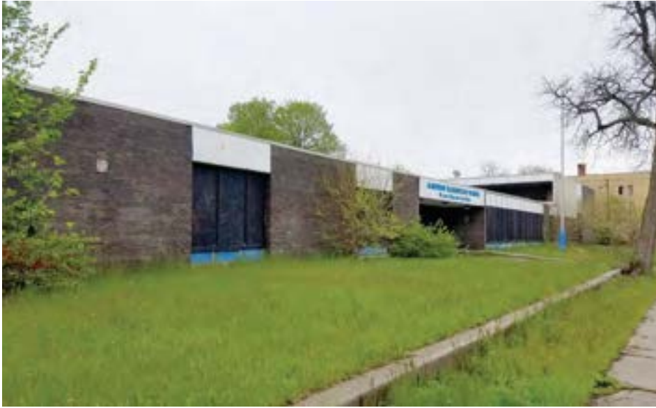
South elevation looking east. The main entrance is visible right of center, and the two-story classroom wing is visible in the background. In contrast to the original 1961 building, which featured continuous glazing, the 1964 unit (foreground) features smaller windows alternating with dark brick walls.
