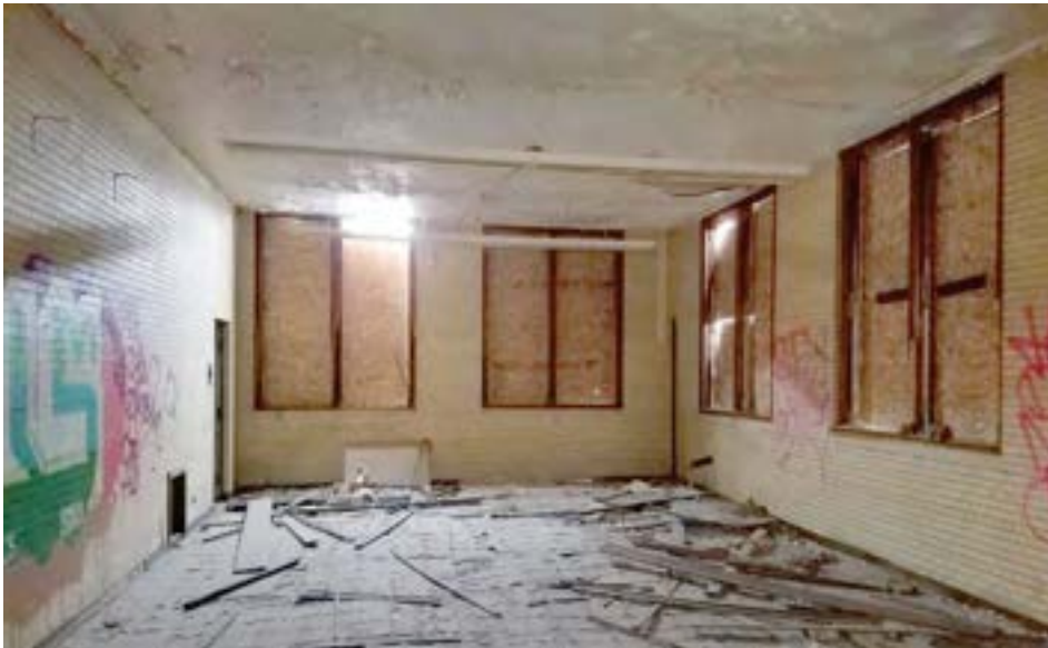
The "play room" is a large auxiliary space located behind the auditorium. Parker has four such spaces clustered in the north wing.
