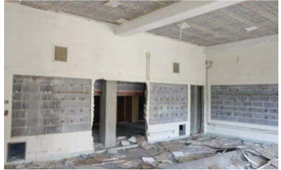
Classrooms in the 1940/1950 west addition are austere, with simple concrete block construction. The rooms feature high ceilings and large windows. Holes in the walls created by scrappers reveal the concrete frame structure.
