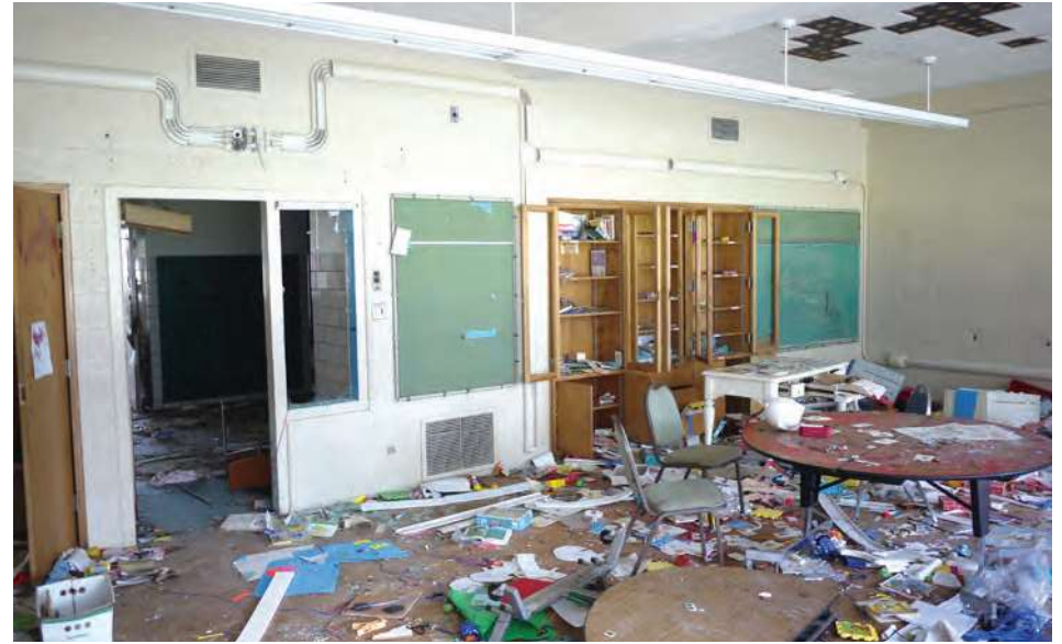
A typical classroom features simple painted CMU walls, acoustic tile ceilings, simple wood cabinetry, and vinyl tile floors. Windows adjacent to doorways admit natural light into the main corridors.
