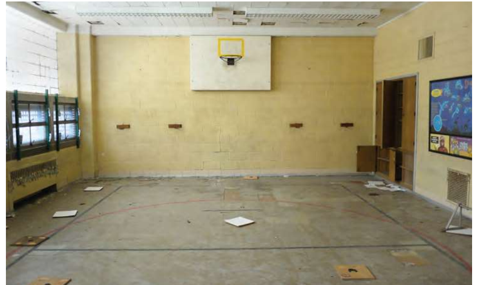
A makeshift gym occupies a standard 22x30' classroom space. Healy lacks large shared spaces like a gym, auditorium, or cafeteria; these were to be included in the unbuilt addition.
