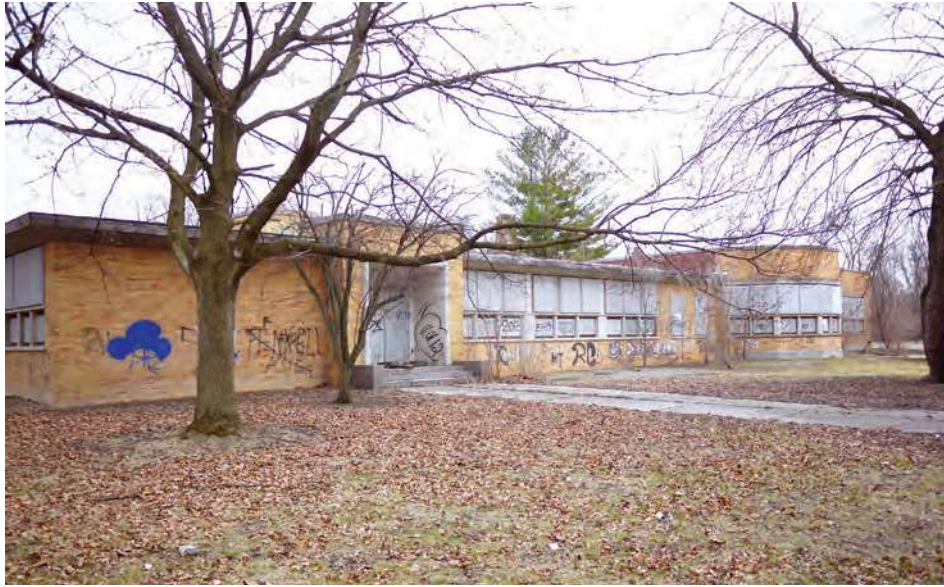
The west facade of the school, showing the original 1924 unit and the 1955 addition. The re-clad original unit includes the large kindergarten bay window and the portion behind it.
