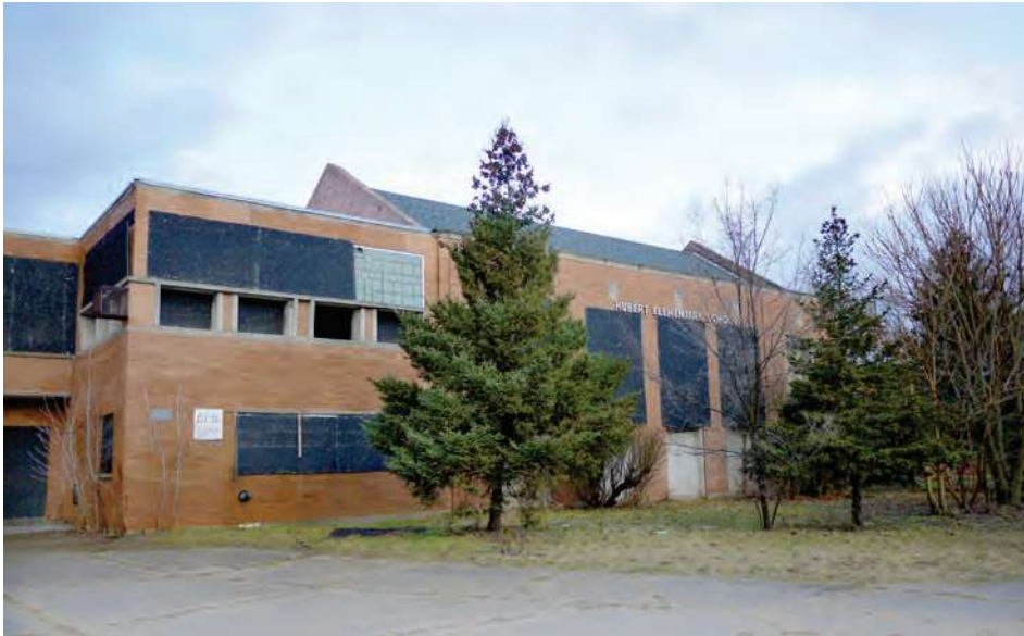
The main street elevation showing the 1930 gym (on right, with gable roof) and 1953 2-story classroom addition. The 1920s, 1930s, and 1950s units have three different architectural styles.
