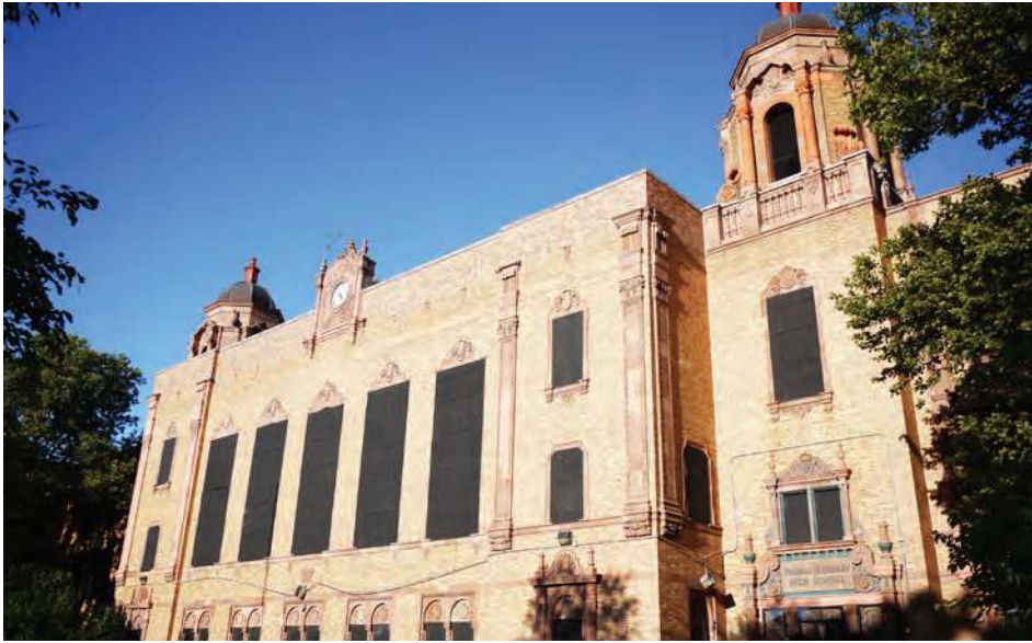
East (main) elevation of the original school building, highlighting distinctive towers and ornate terra cotta details.
