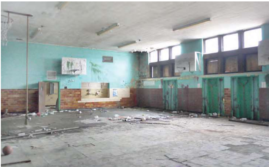
The gym/cafeteria gym looking towards the serving window. The current kitchen is a later update that occupies what was formerly the north entrance vestibule.
