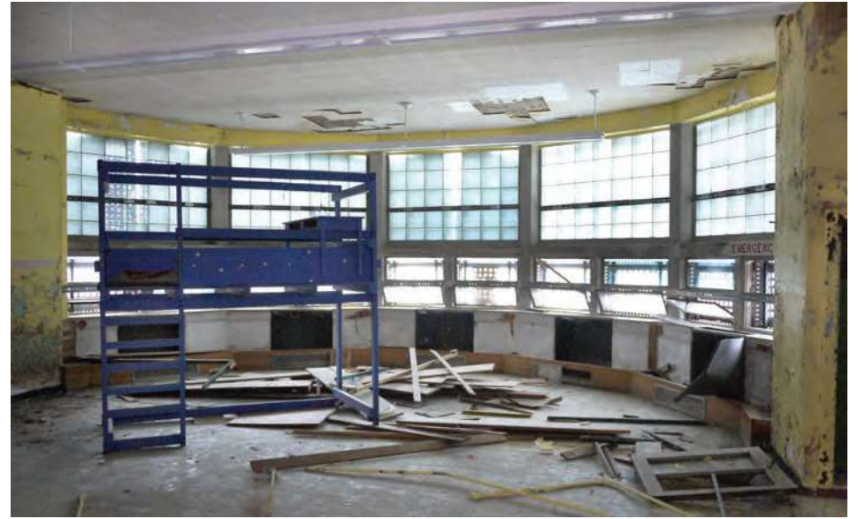
The kindergarten bay has a layout typical of schools from the 1920s. The windows were replaced with glass-block and operable steel-frame style to match the 1955 addition.
