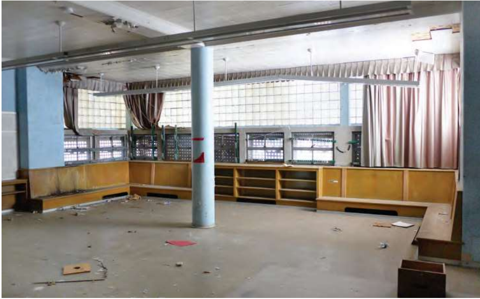
The kindergarten features a glass-box extension that allows daylight from three sides. The “temporary auditorium” space also has this feature.
