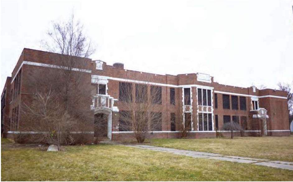
The main (south) facade of the original 1925 wing.
