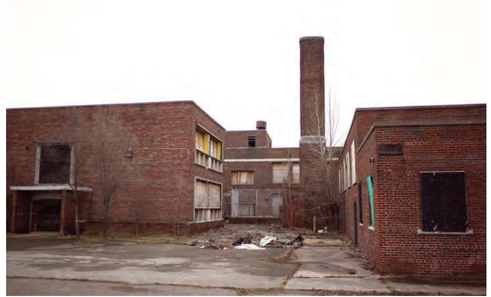
Courtyard and modern-style 1959 wings viewed from the north. The 1959 wings featured large glass-block ribbon windows, a contrast to traditional windows in the original unit.
