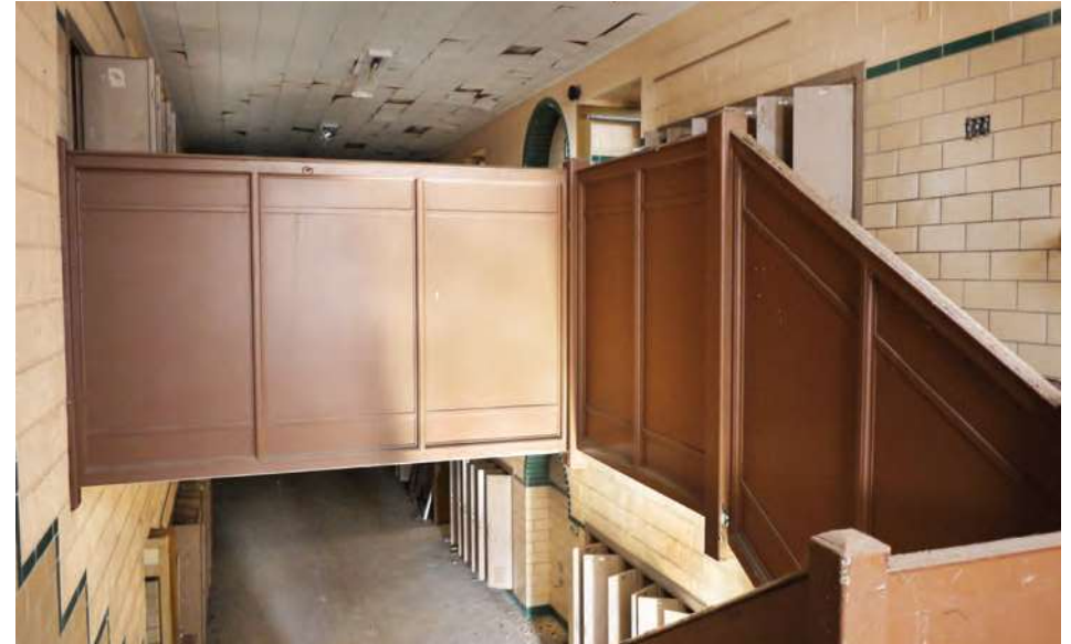
The south stair features painted steel panel railings.
