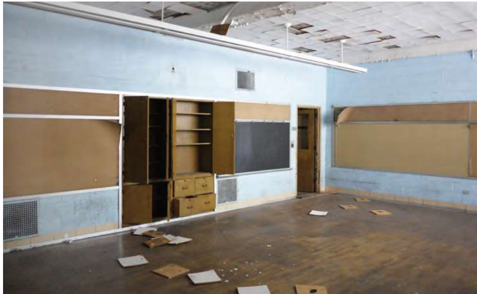
A typical classroom, showing finishes in excellent condition.
