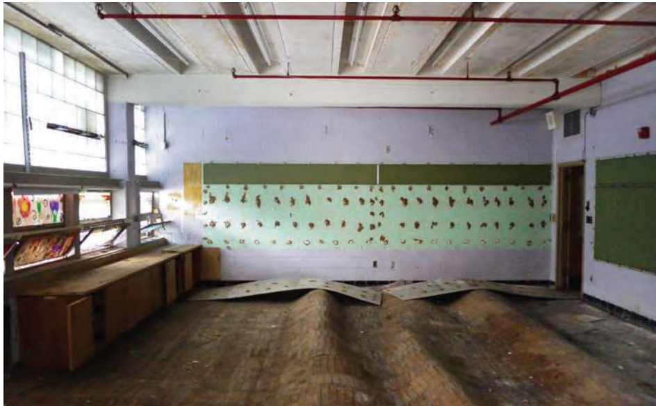
Classrooms are brightly-lit thanks to the wall-to-wall windows. Partition walls can be easily added or demolished thanks to the school's flexible post-and-beam structure.
