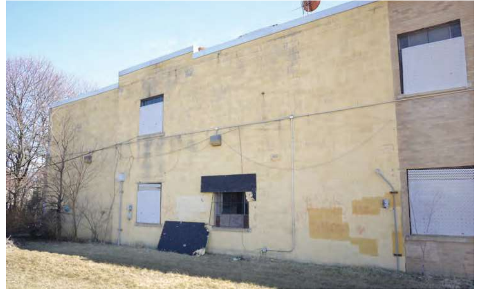
The north half of the school's west elevation is only roughly finished with CMU, to accommodate a large planned addition that was ultimately never built.
