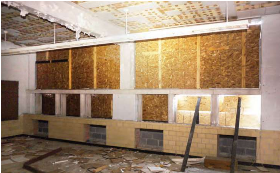
Typical window configuration and concrete block finishes in modern 1959 classrooms.
