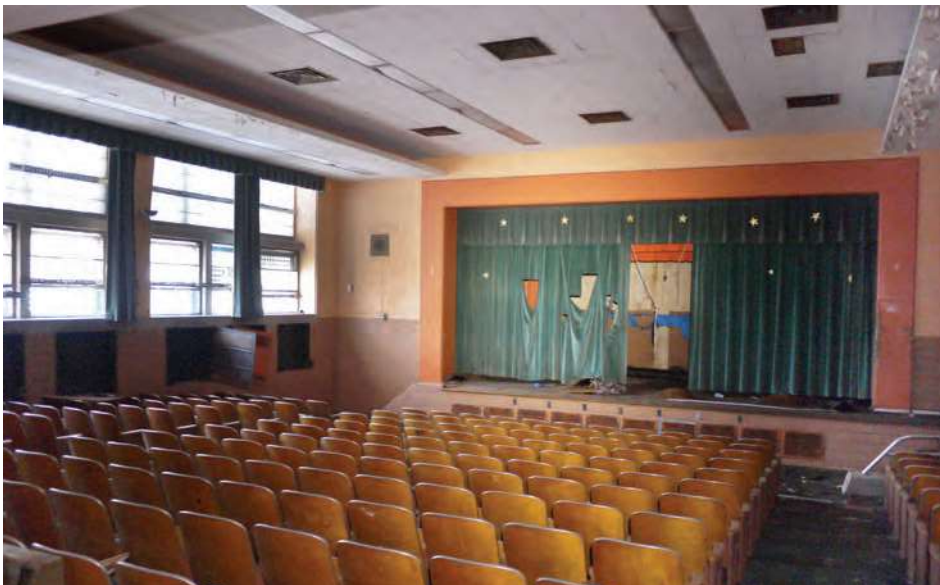
The simple concrete-block auditorium was built as part of the 1955 addition. It is in good condition, with seats and finishes intact.
