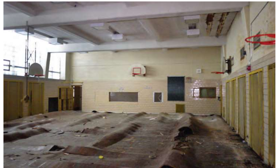
The gym/cafeteria is a 40x60' box with 16.5' ceilings, standard for elementary schools. There is an attached kitchen with small serving window located at the south end (visible on rear wall)
