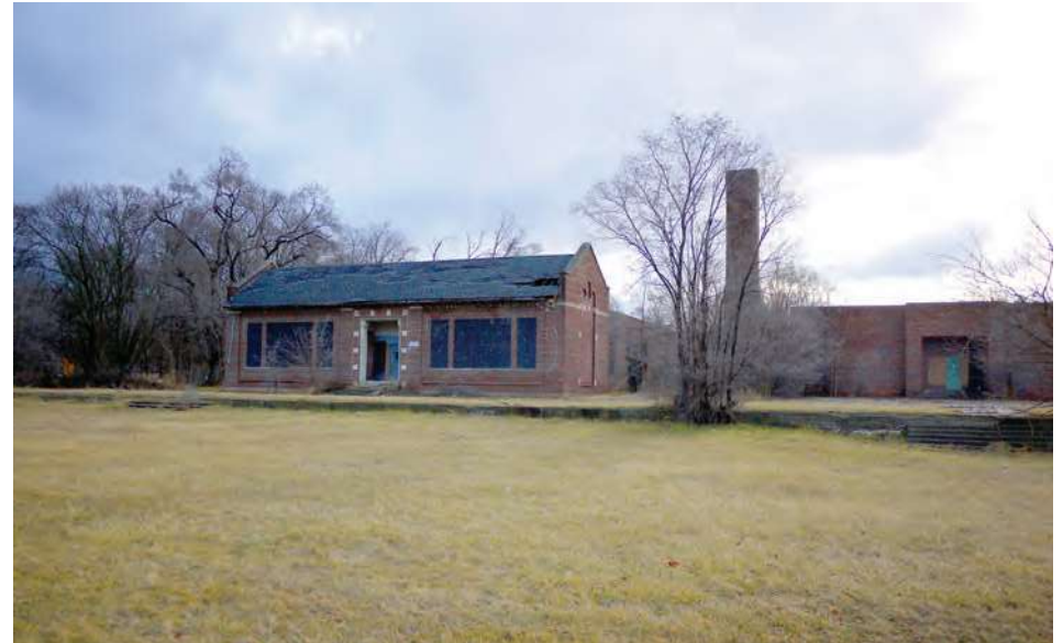
Original 1925 unit, viewed from the spacious school yard behind the school. The 1-story 1930 expansion is visible to the right of the frame. Damage is visible on the sloped roof.
