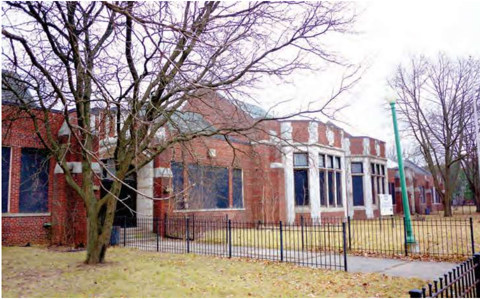
Primary west elevation, featuring symmetrical design anchored by double-bay windows.
