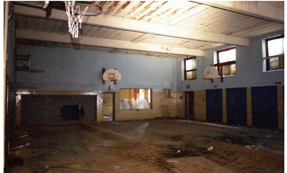
Gymnasium and kitchen serving window.
