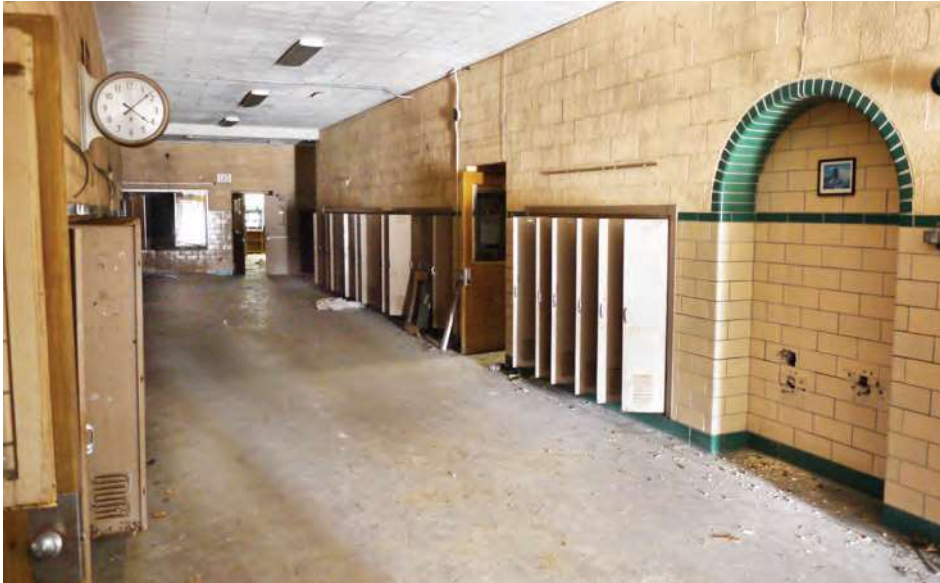
This photo captures the entire length of the main first floor corridor. Hallways feature a combination of CMU and glazed block, with green glazed tile accents.
