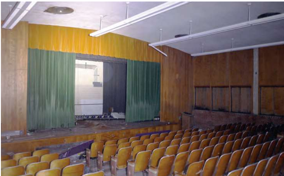
The small auditorium has a unique wood panel finish, including sliding blackout panels at the windows. There is water damage to the stage area, but the space is otherwise in good condition.
