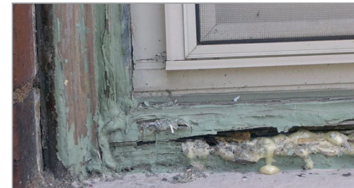
Windows And Window Sills
