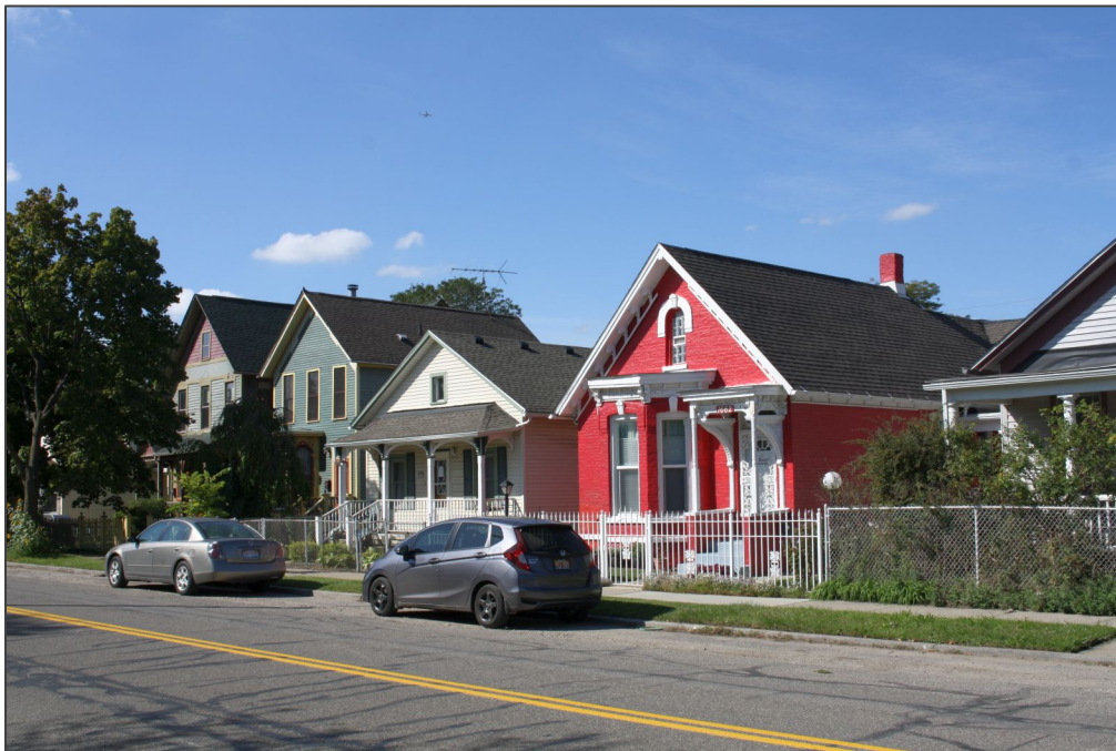
Figure 7. Houses along the north side of Bagley Street
