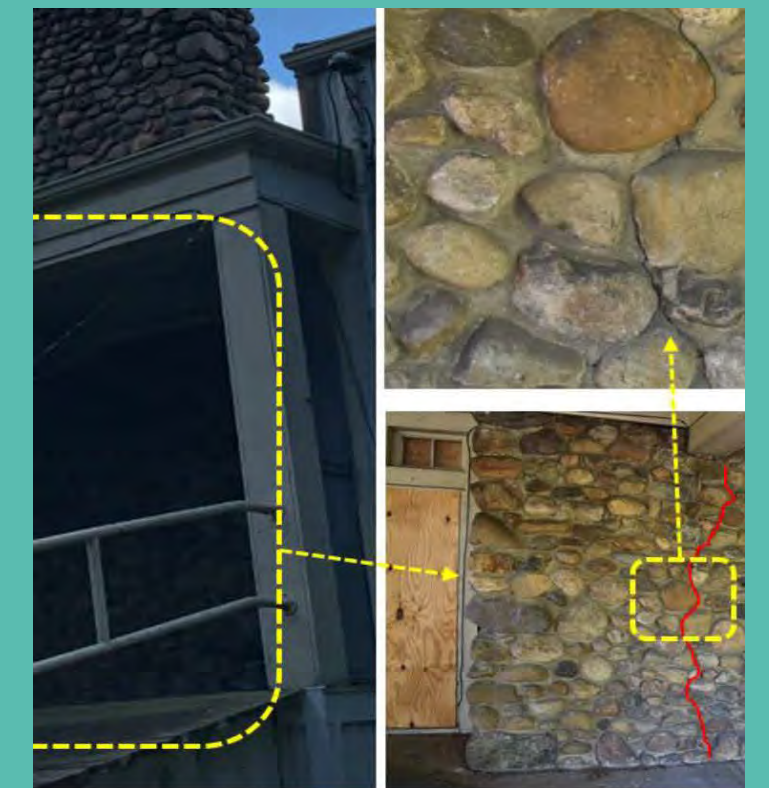
portion of the fieldstone chimney and vertically oriented crack
