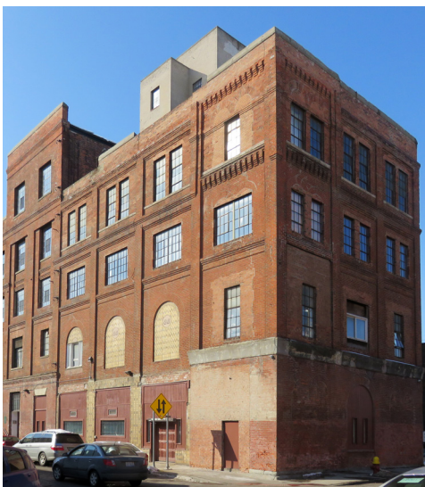
Converted loft apartments are the most common form of housing the Core Market. Photo: Kramer Design Group
