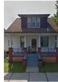
1.5 story single family wood construction built ca. 1920s (area varies)
