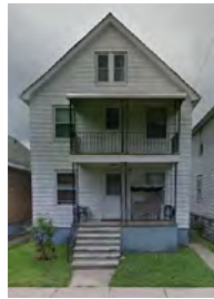
2.5-story duplex wood construction built ca. 1920s 1500 - 3000 sf
