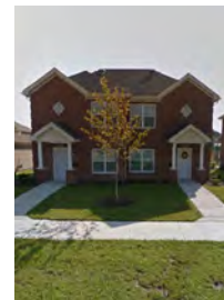
2-story duplex brick construction built 2011 (area unknown)
