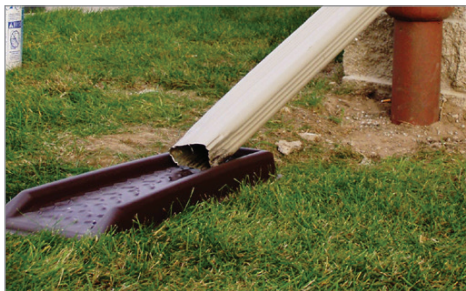
Downspouts should be directed to a lawn area or a rain garden.
