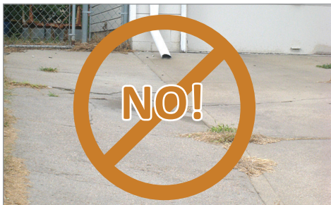
Downspout should not be directed to impervious areas as depicted in this example. Here stormwater flows down the driveway to the street. The discharge can also cause an icing hazard.
