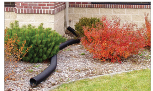
Simple techniques like elbows, extensions, or rain chain/cascading designs can help direct stormwater away from the foundation, property, and on to lawn areas.
