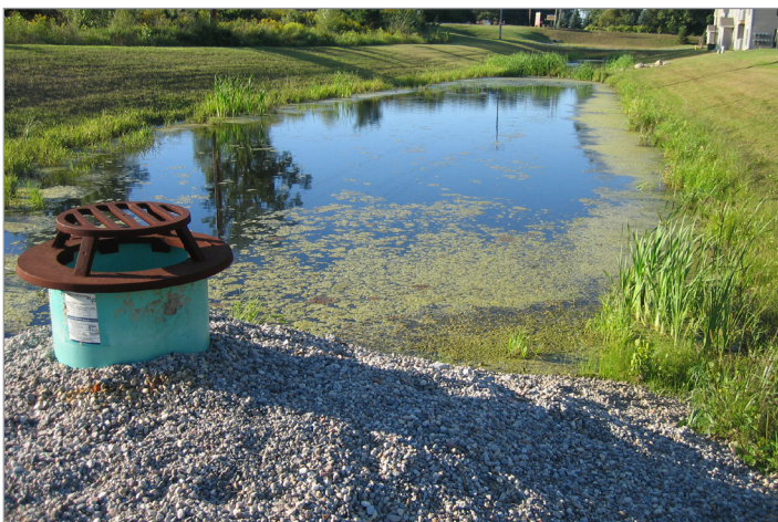
Retention basin with outlet riser in the forefront of the photo
