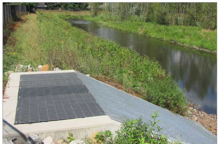
Retention basin with inlet structure in the forefront of the photo
