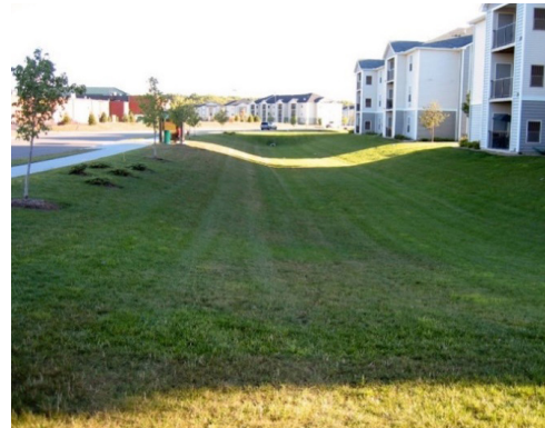
Traditional Dry Detention Basin
