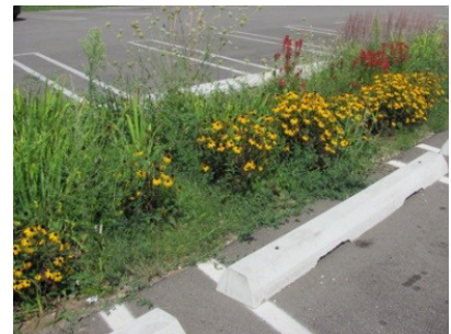
Bioretention between Parking Lot Aisles
