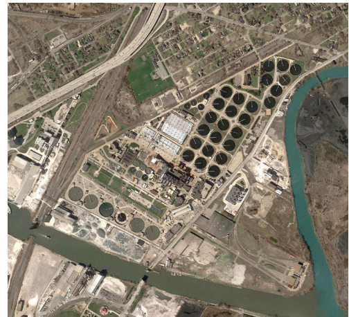
Detroit's Wastewater Treatment Plant
