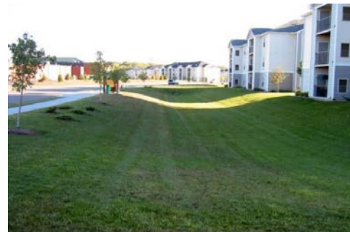
Dry Detention Basin
