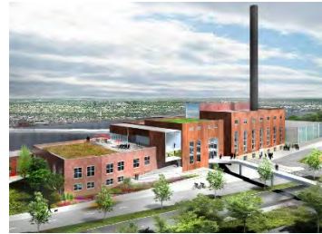
Beloit Powerhouse Beloit, WI
