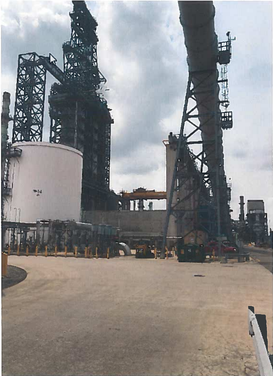
View of Coke Pit Wall/Coker/Conveyor from Northeast
