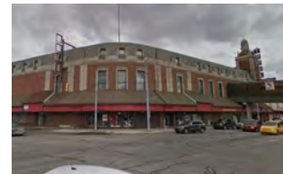
Tower Center 15400 Grand River
