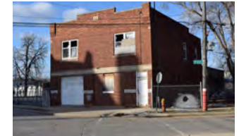
Former Fire Station & Redford Village Hall (1921) 22050 Argus
