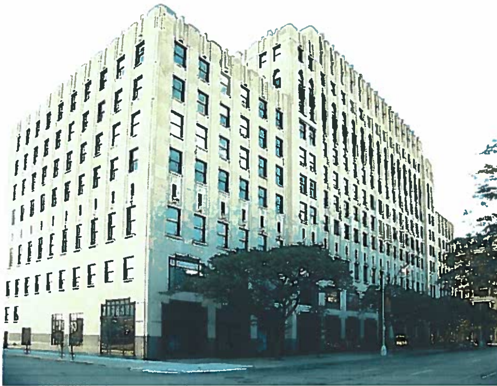
Albert Kahn Building
