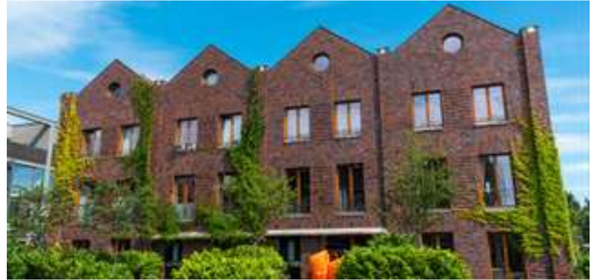
f. Adaptive reuse of existing structure
