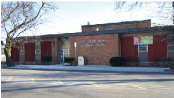
Chandler Park Branch Library
