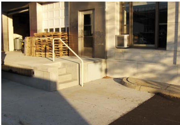
Asphalt/Repaving at Main Library
