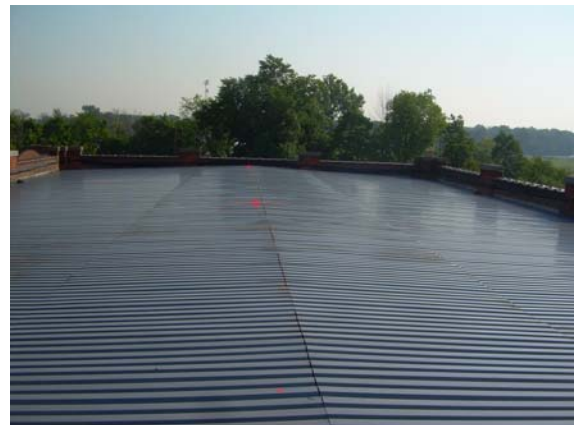
Belle Isle Maintenance Garage Roof 2007
