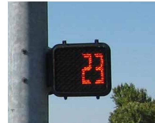
PEDESTRIAN COUNTDOWN TIMERS and reasonable crossing times to make it easier to cross at traffic signals.
