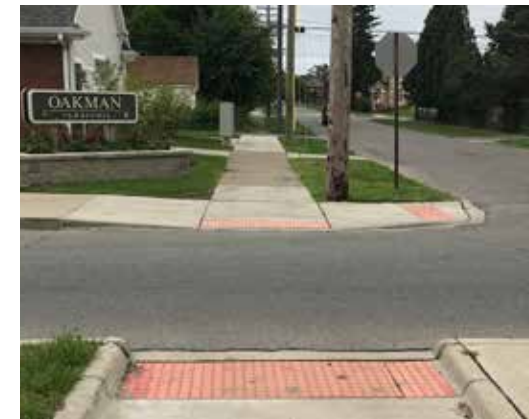
ADA-COMPLIANT CURB RAMP s at every crossing so that people of all abilities can get around.
