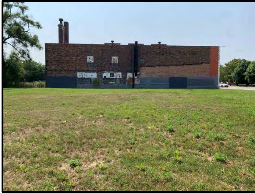
VIEW OF SUBJECT PROPERTY – FACING SOUTH
