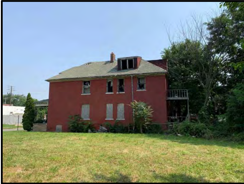
SUBJECT BUILDING – FACING EAST
