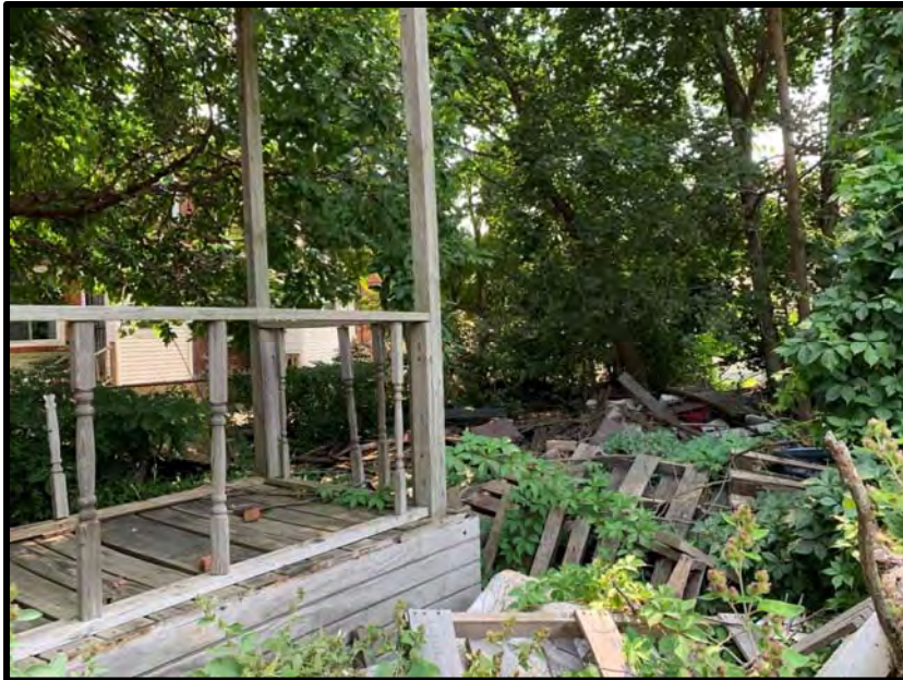
EXTERIOR OF SUBJECT PROPERTY (INACCESSIBLE)
