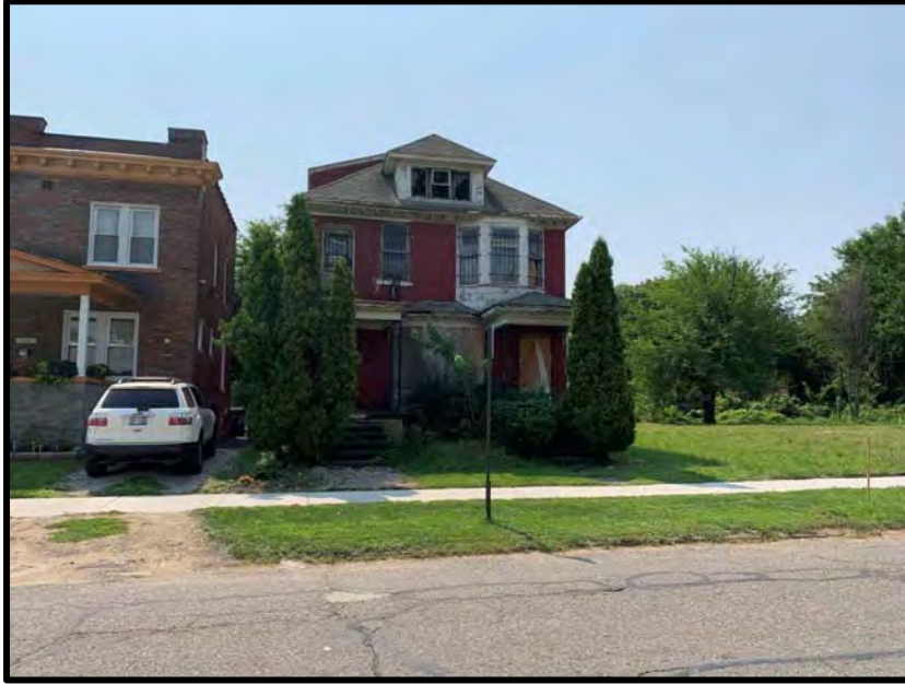
SUBJECT BUILDING – FACING SOUTH
