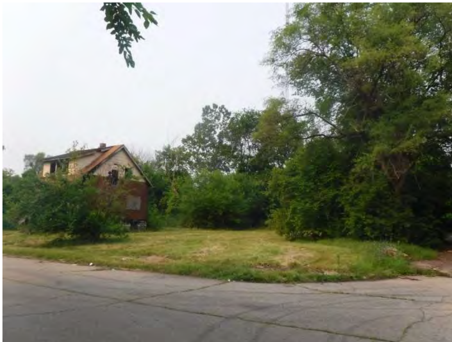
Photo 14: Looking southwest at an overgrown and vacant formerly residential area along Ward Avenue in the northeast portion of the Subject Property. The dwelling seen at left is located at 14173 Ward Avenue and was marked condemned as dangerous and unsafe.
