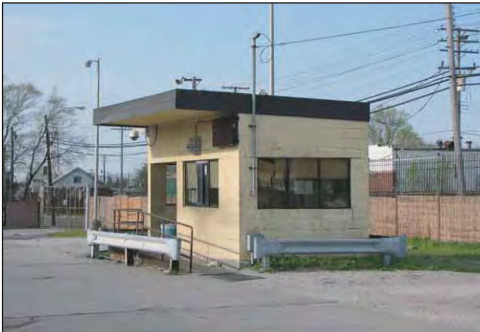
Figure 3. -1. Dispatch House East and North Elevations
