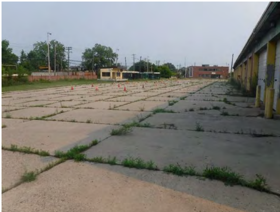
Photo 38: Looking northwest at the concrete paved area west of the Main Building at the Subject Property. The former Dispatch Building is seen at left in the background, and the Terminal Building is seen to its right. Both are located along Schaefer Hwy.
