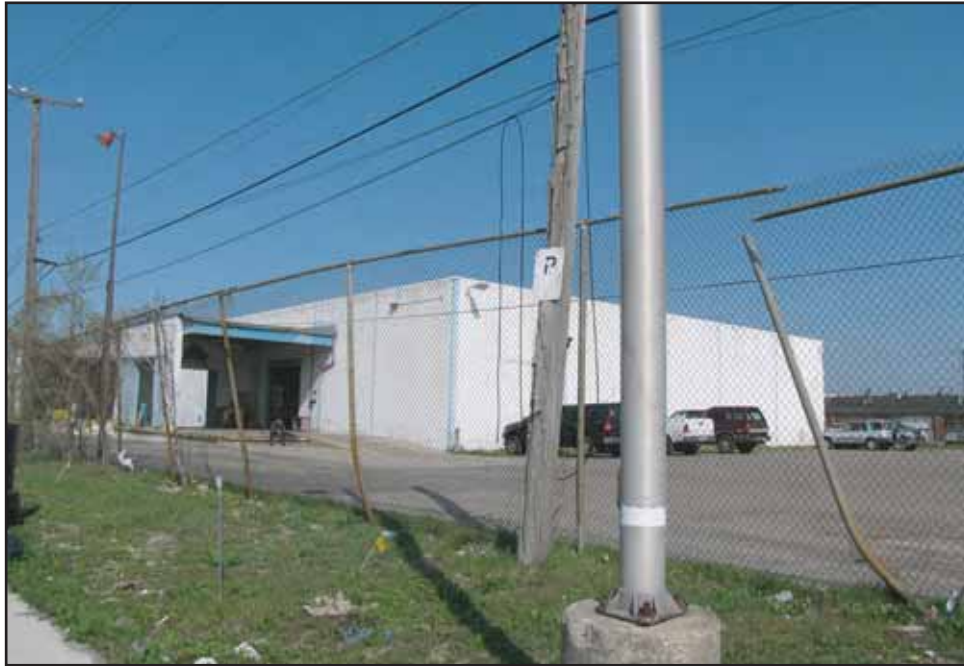
Figure 3.0-4. Section of Chain-link Fence at Coolidge Terminal
