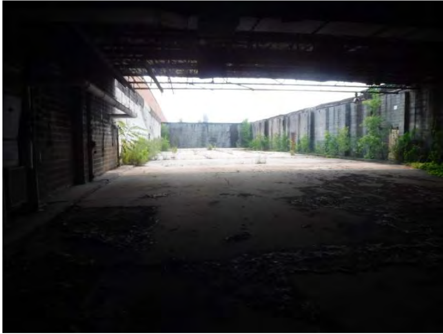
Photo 31: Looking east at the fire damaged portion of the former coach storage area within the Main Building.
