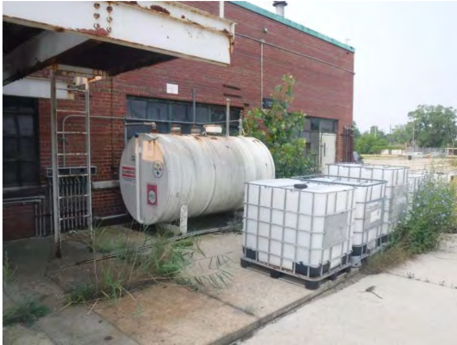
Photo 33: Looking southwest at a 1,500-gallon antifreeze aboveground storage tank and several empty 250-gallon and 275-gallon totes stored north of the gas house portion of the Main Building.
