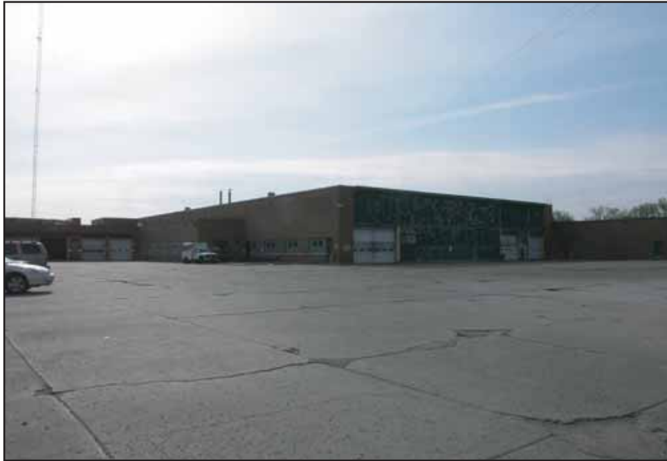
Figure 3.3-1. Bus Maintenance Garage West and North Elevations
