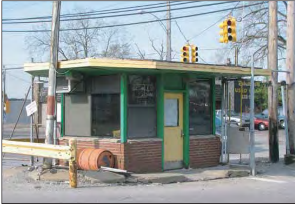
Figure 3.5-1. Gate House North and East Elevations
