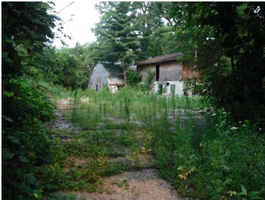
Photo 44: Looking northwest at a former electrical shop located at 13200 Intervale Street which adjoins the Subject Property to the northeast.
