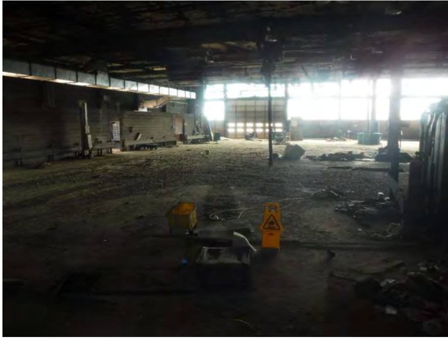
Photo 25: Looking northeast at sand from an unknown location which was present on the concrete floor throughout the eastern portion of the maintenance area of the Main Building.
