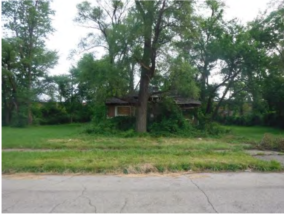
Photo 5: Looking north at a former residential dwelling located in the southwestern portion of the Subject Property along Compass Street. This dwelling is now abandoned and in severe disrepair, and was not physically entered.
