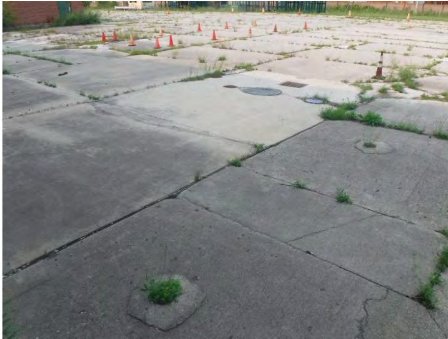
Photo 39: Looking southwest at the location of a waste oil underground storage tank to the west of the maintenance area of the Main Building.
