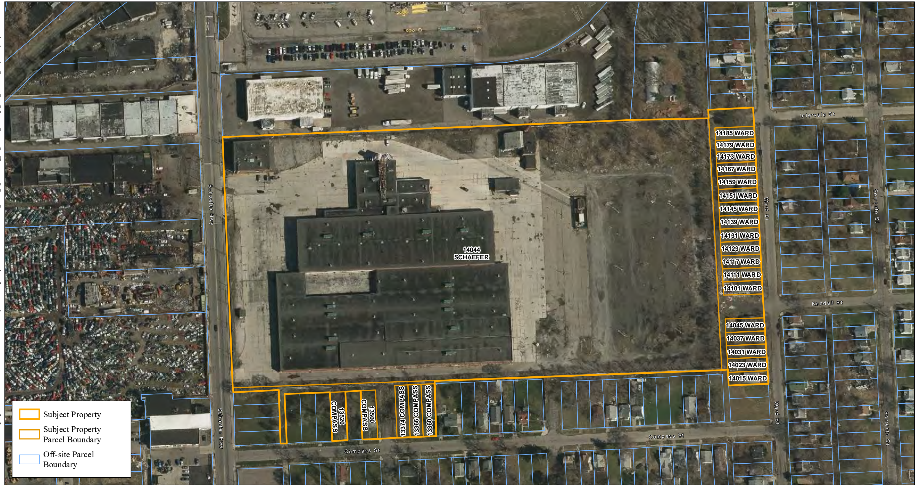
Figure 2 Subject Property Former Coolidge Bus Terminal and Vicinity 14044 Schaefer Hwy Detroit, MI 48227 Detroit Building Authority
