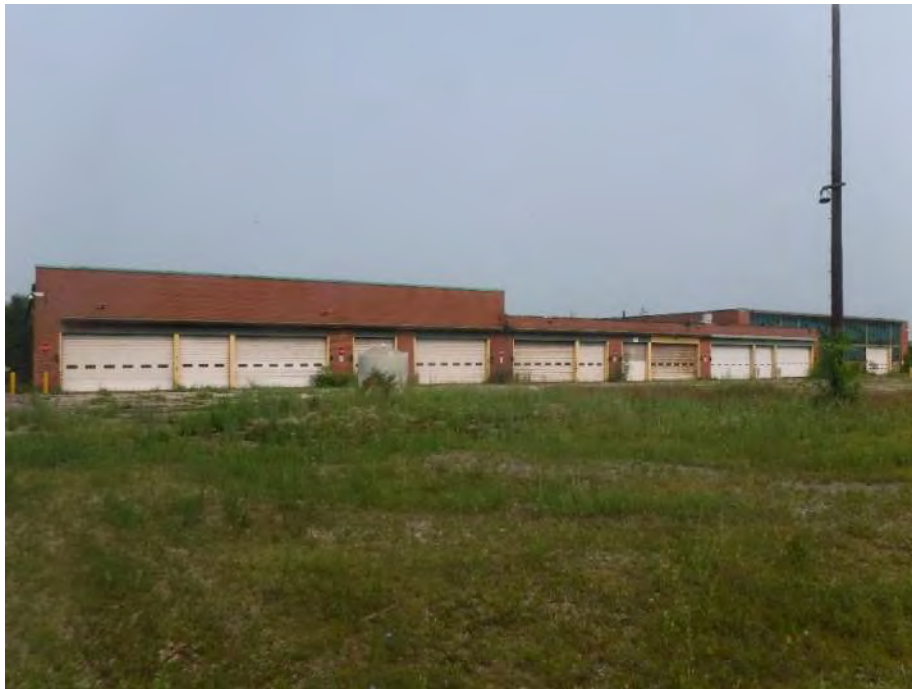
Photo 2: Looking northwest at the rear side of the former Coolidge Bus Terminal building, which was originally constructed in 1928 as a streetcar maintenance facility and was converted to bus maintenance and storage in 1947.
