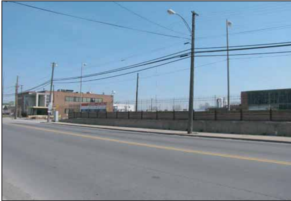
Figure 3.0-2. Coolidge Terminal Property West Wall
