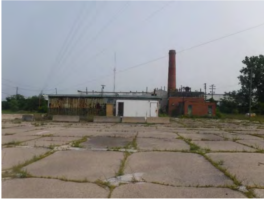
Photo 3: Looking north at the former Fare Box Building (left) and Heating Plant Building (at right adjacent to stack). Guy wires for the onsite antenna tower are also visible.
