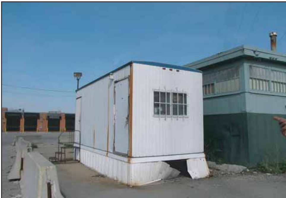
Figure 3.0-5. Temporary Office Trailer East and South Elevations
