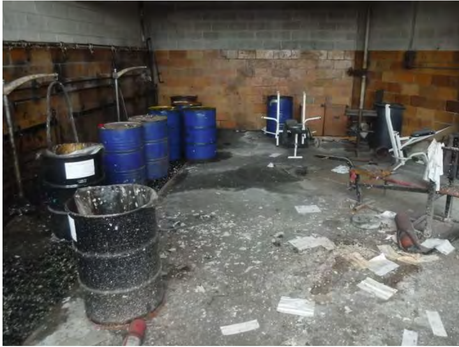
Photo 29: Looking northeast at the pump room in the western portion of the maintenance area within the Main Building. Various lubricants and waste remained within 30 and 55-gallon steel drums in this area.
